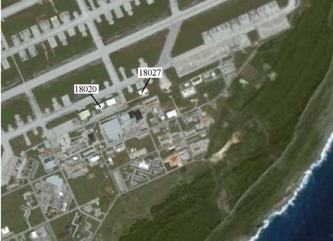
Figure 1.4. Aerial view of a portion of Andersen AFB showing Buildings 18020 and 18027.
