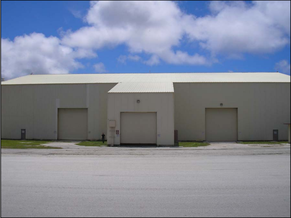
Figure 3.9. North-northwest-facing view (south or rear elevation) of Building 18020.
