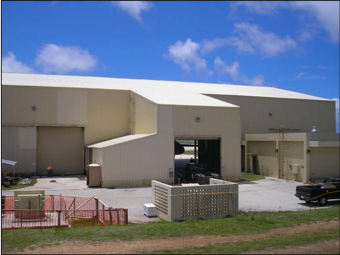
Figure 3.10. North-facing view (south or rear elevation) of Building 18027.
