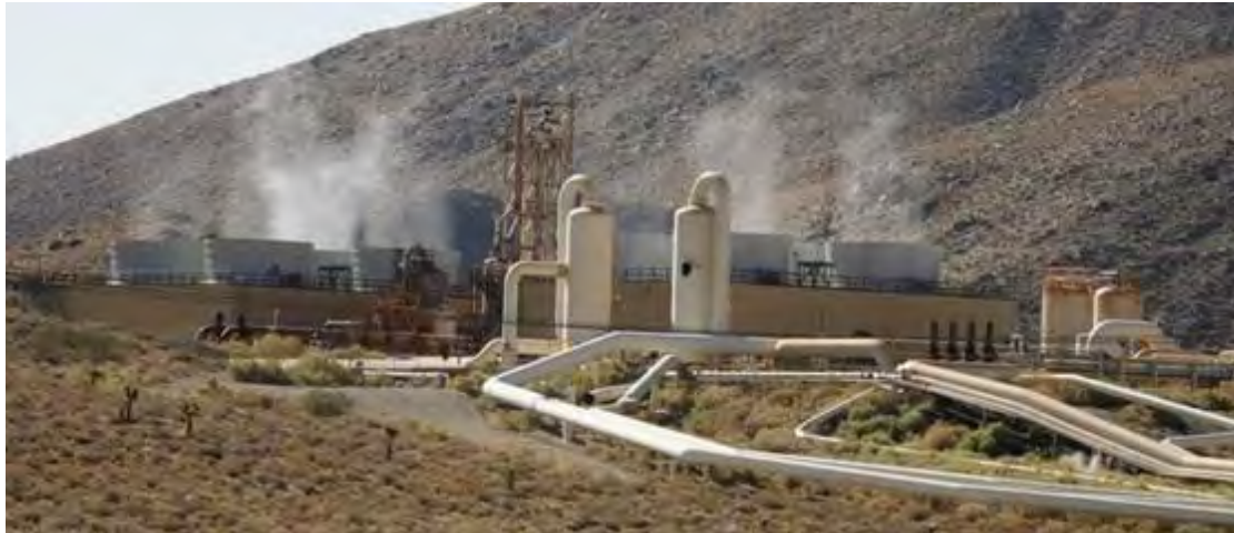
China Lake Geothermal Power Plant, 270 MW, since 1987
