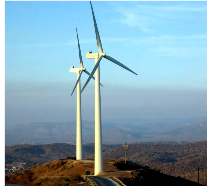
Guantanamo Bay Wind Farm, 3.8 MW
