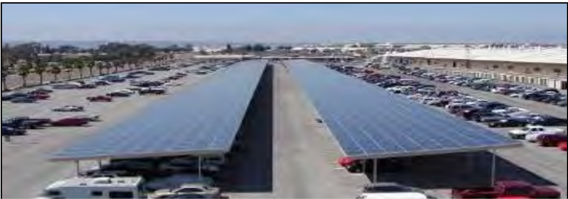
North Island Solar Power array on parking garage, 1 MW
