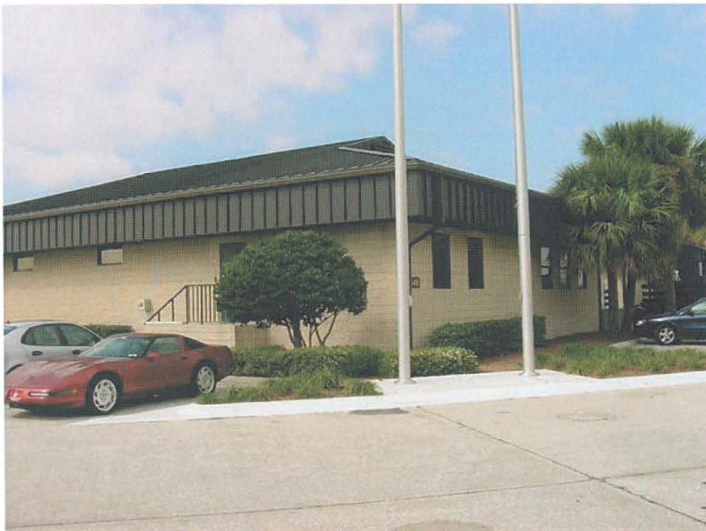
Photograph 10: Building 546 looking to southwest
