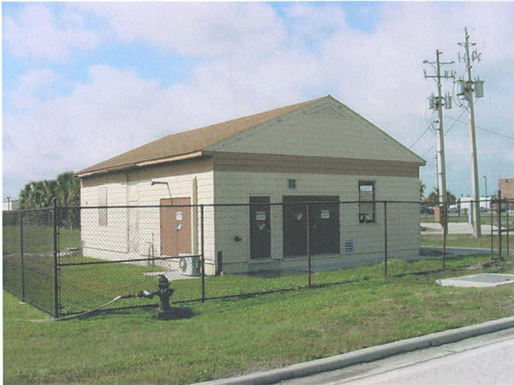
Photograph 11: Building 927 looking to southwest
