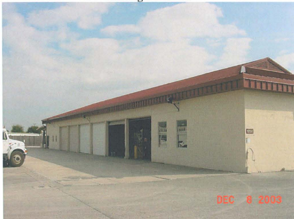
Photograph 14: Building 1050 looking southeast
