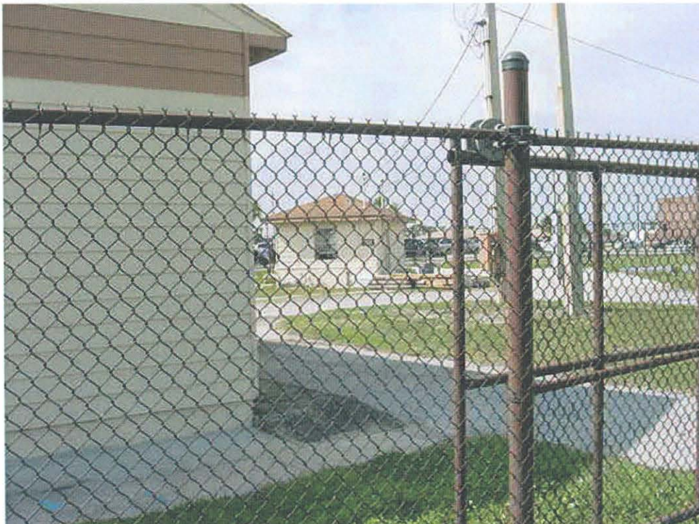
Photograph 12: Building 928 looking to southwest
