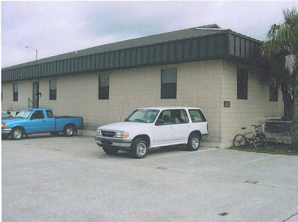
Photograph 3: Building 531 looking towards northeast
