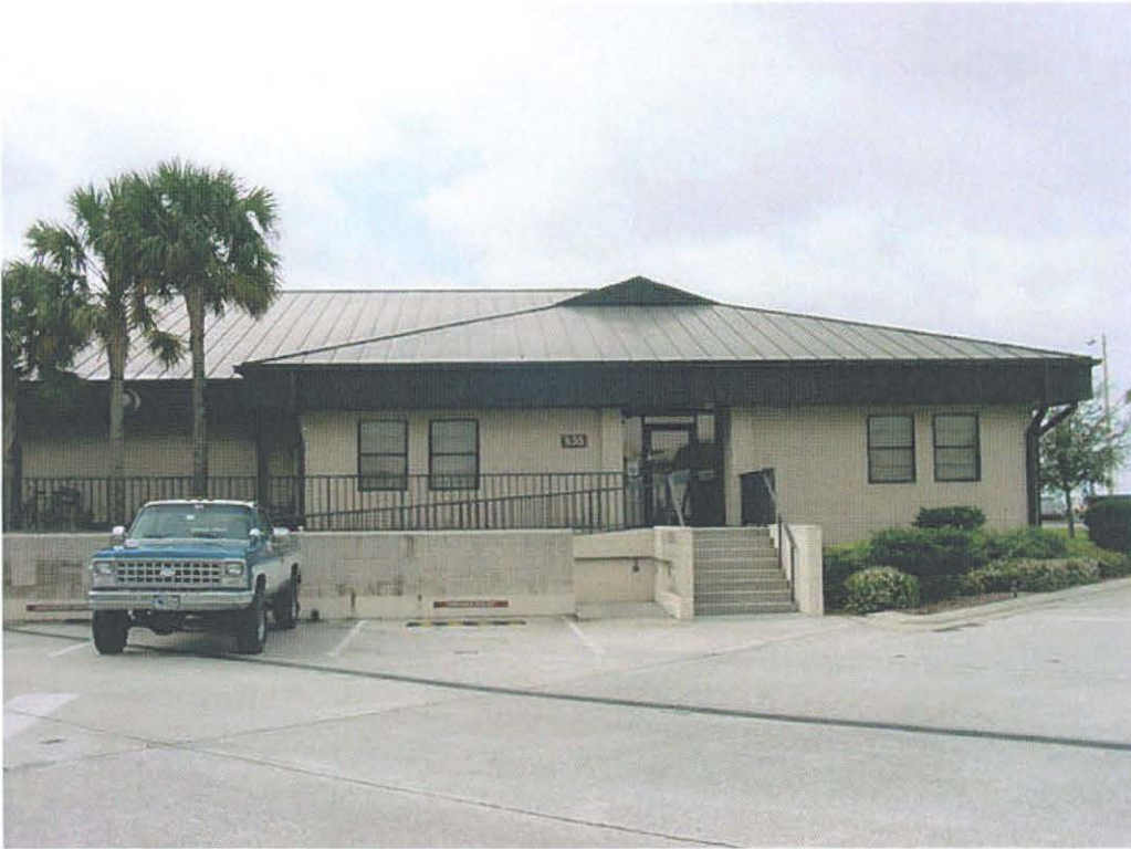
Photograph 5: NAVCENT/MARCENT (Building 535) looking from east
