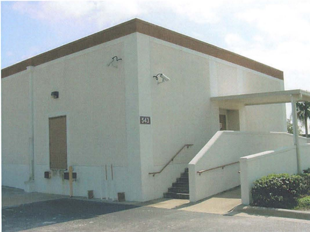
Photograph 9: Building 543 looking to southeast
