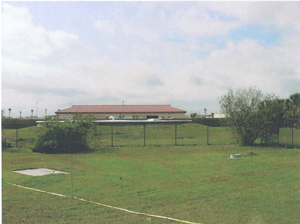
Photograph 1: Water Tank (Building 95)
