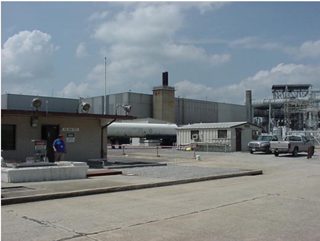
Photo 3. Proposed Fuel Laboratory Site, looking north.
