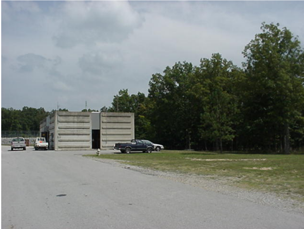
Photo 5. Proposed Bromine Storage Trailer Building Site, looking north.
