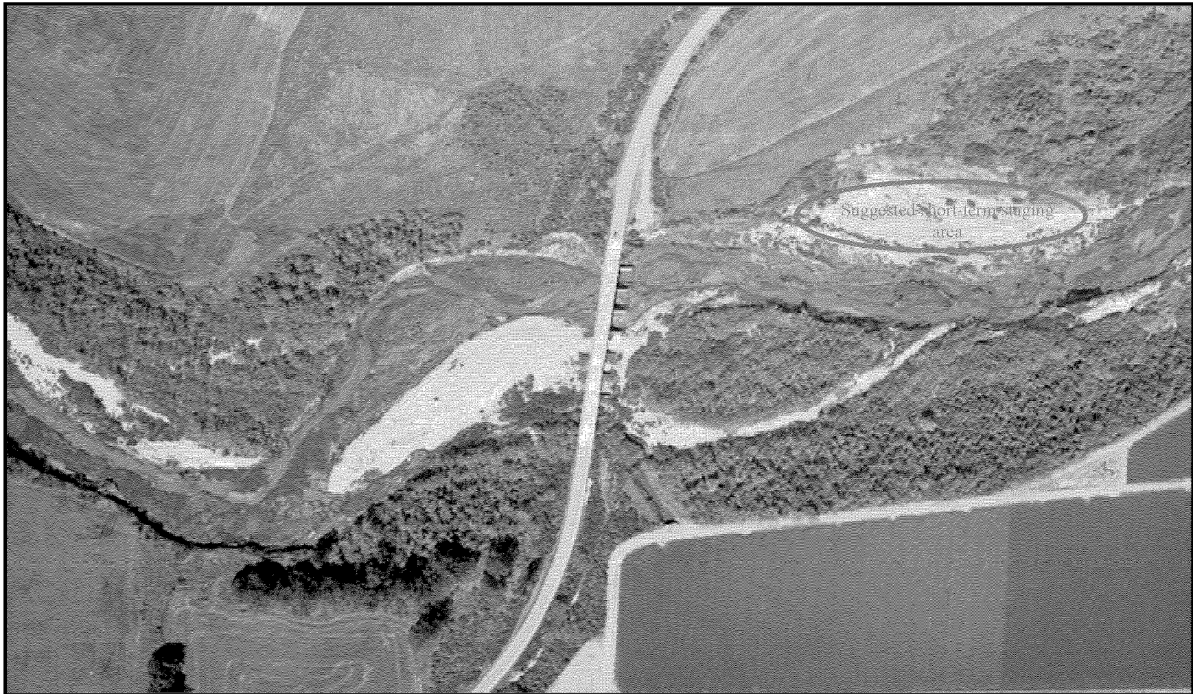
Figure 2-6. Aerial view of 13 th Street Bridge vicinity and suggested short-term staging area in upstream unvegetated sandbar for proposed retrofit project.
