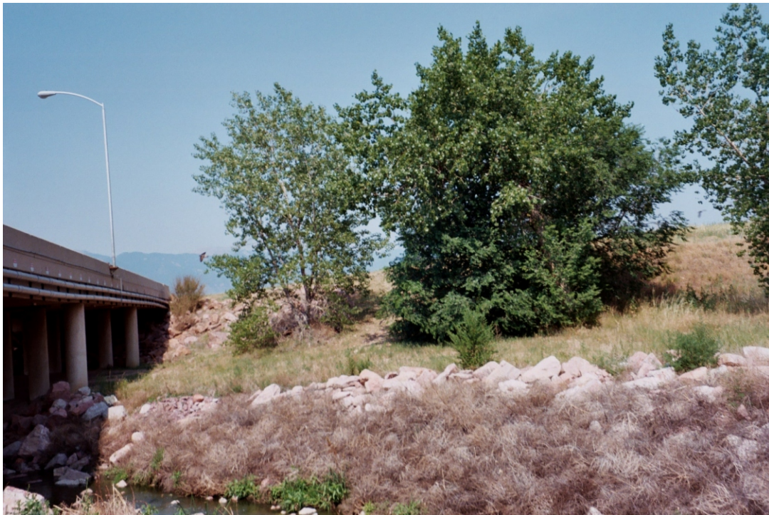
Photo 6 West Bank of the East Branch of Sand Creek
