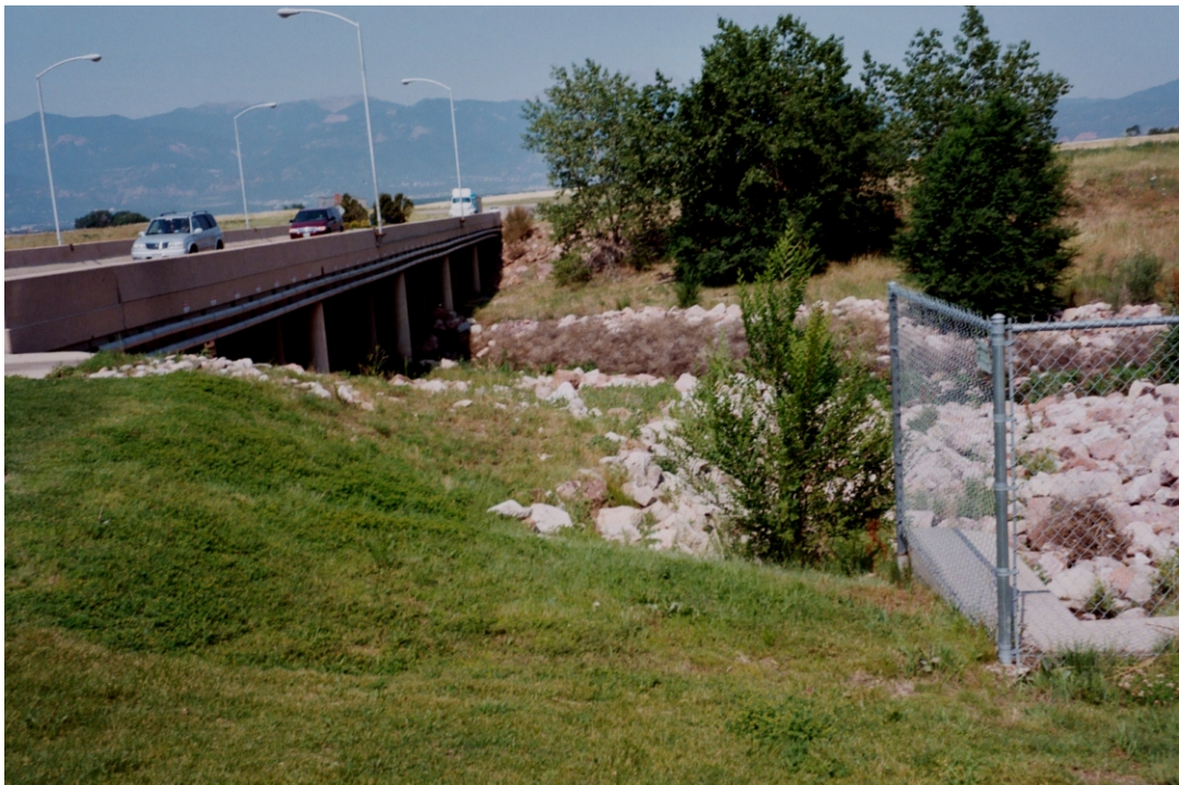
Photo 4 Existing Bridge over East Branch of Sand Creek near West Gate
