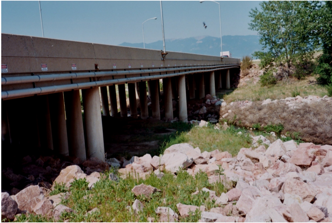
Photo 5 Closeup of Existing Stewart Ave Bridge near West Gate
