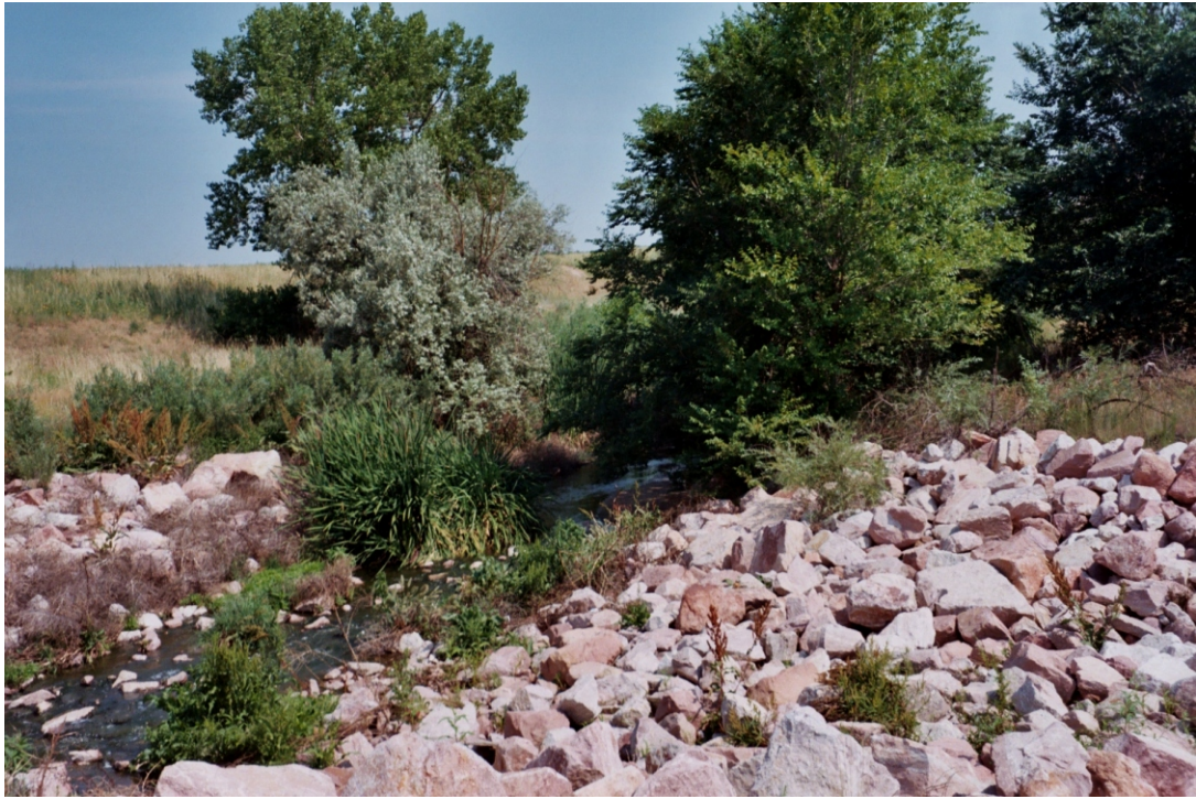
Photo 7 East Branch of Sand Creek Just North of Stewart Ave Bridge
