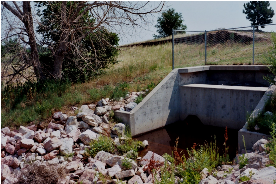
Photo 8 Outfall 1 at East Branch of Sand Creek Near West Gate
