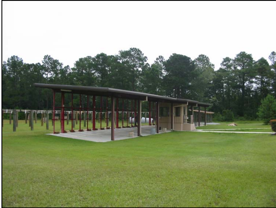
View of existing CATM Range structure and target supports
