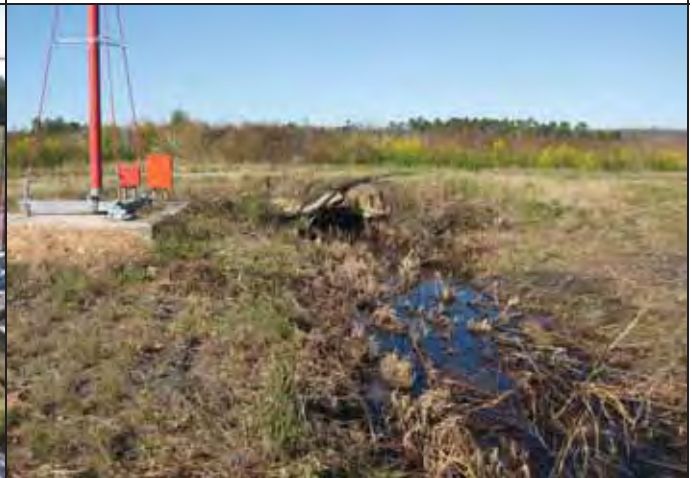
Culvert under perimeter access road
