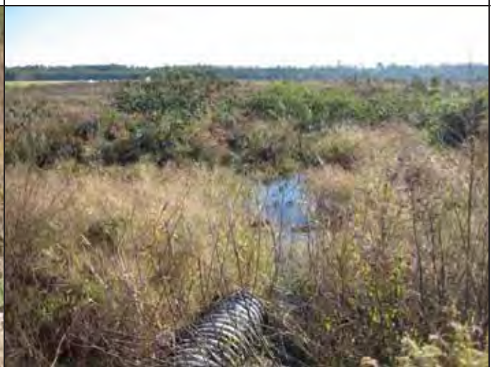
Culvert draining into South EOR wetlands
