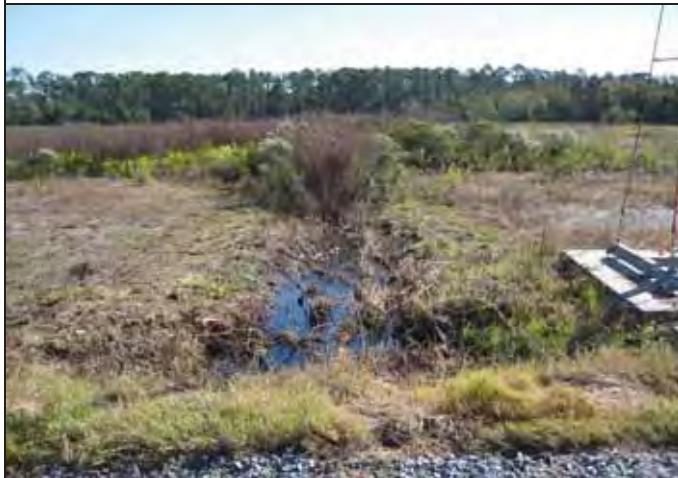
Culvert under perimeter access road
