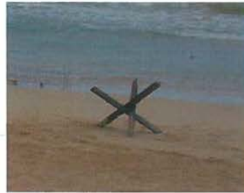
Figure 3. Structural hedgehogs measuring 1 m x 1m x 1m in approximately 1.3-m depths with 10 m spacing.
