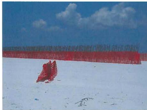
Figure 4. Structural sea urchins are 3 pieces of rebar welded in the shape of a teepee measuring and erected in a row measuring 2m tall, 0.9-m in depth, and 100 m long. (structural sea urchins placed in water will not be wrapped in fencing as shown)
