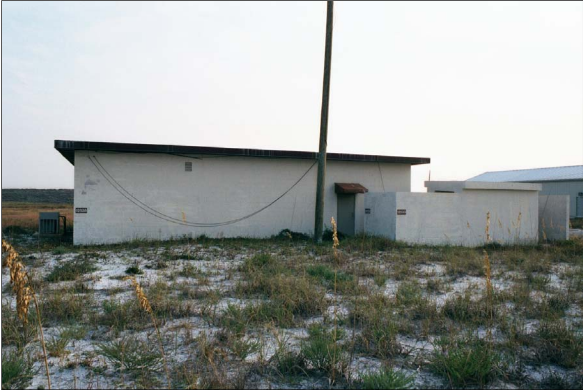
Photo 3. Building 12528 (left) and Building 12533 (right), north elevation.
