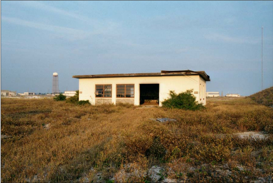
Photo 5. Building 12534, west elevation.
