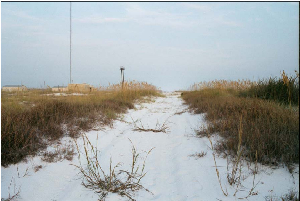
Photo 8. Access road for Building 12588, west elevation. Building 12588 is located on left.
