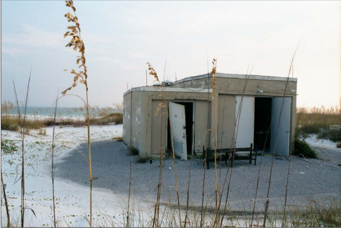
Photo 7. Building 12588, north elevation.
