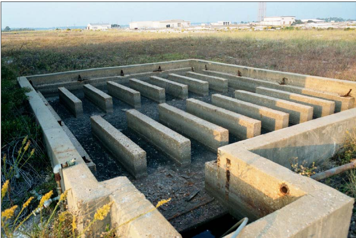
Photo 6. Remains of cooling tower structure associated with Building 12534.
