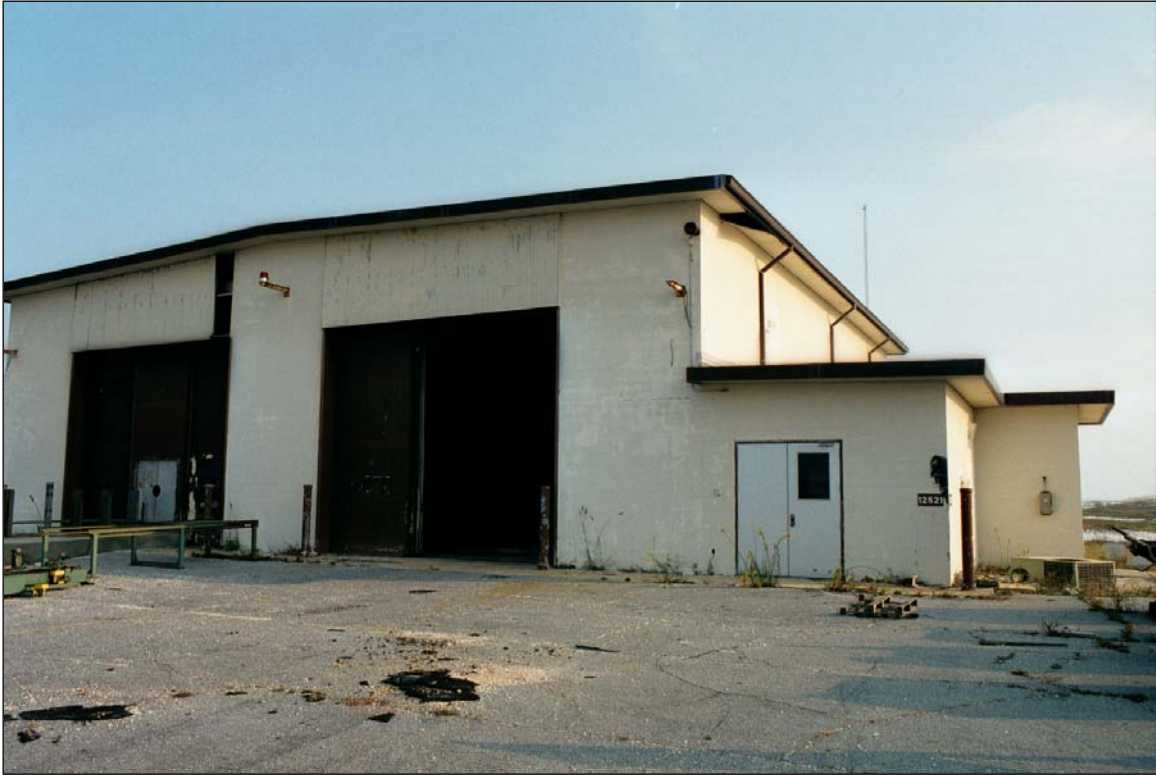
Photo 1. Building 12521, north elevation.
