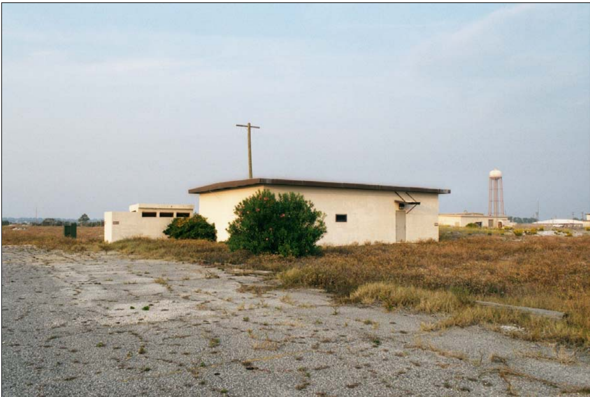
Photo 2. Building 12533 (left) and Building 12528, southwest elevation.
