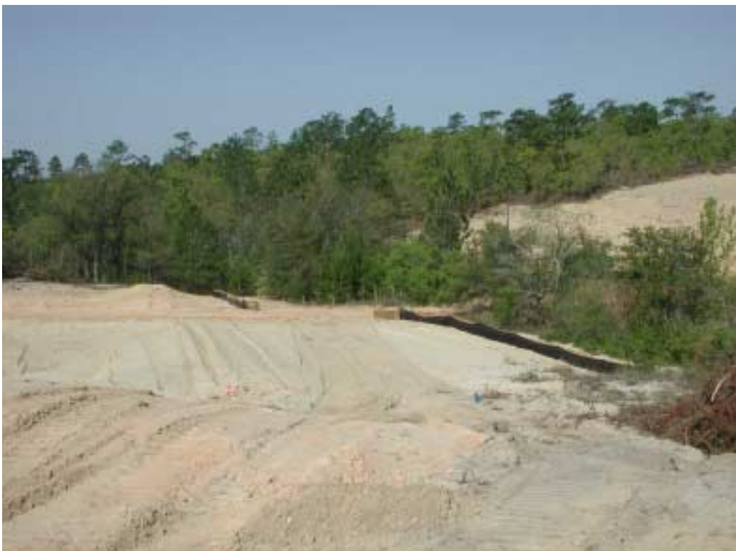
Downrange Impact Area Erosion Control Project (west side of stream)
