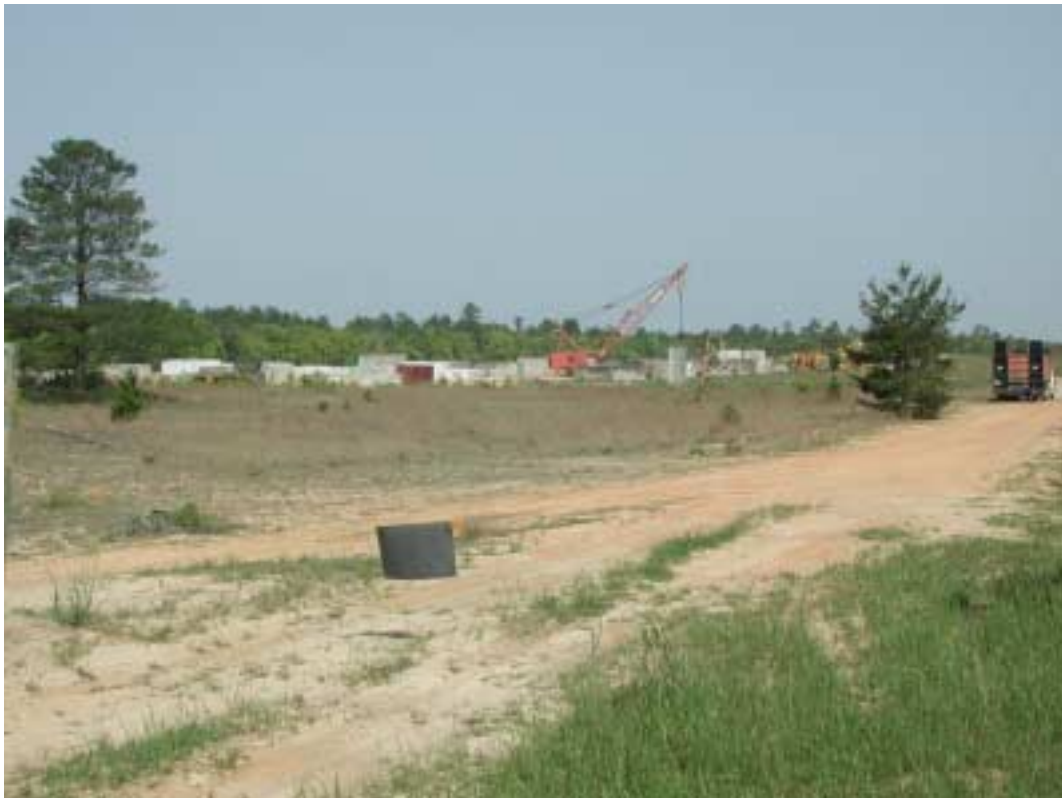
Target Construction Area
