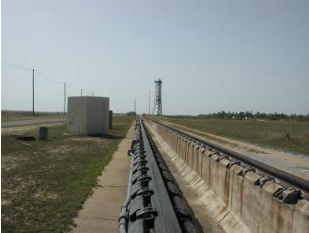
Sled Track: North to South, with observation tower
