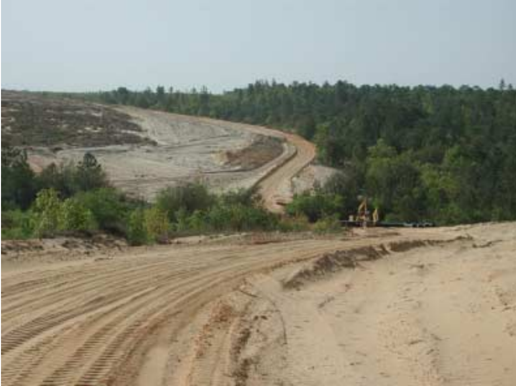
Downrange Access Road and Erosion Control Project
