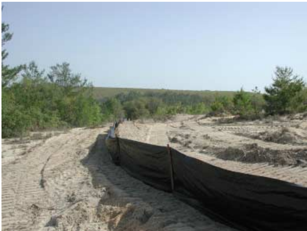
BMPs for Sedimentation Control near Okaloosa Darter Stream (east side of stream)
