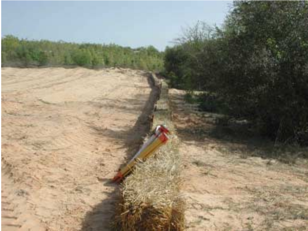
BMPs for Sedimentation Control near Okaloosa Darter Stream (west side of stream)
