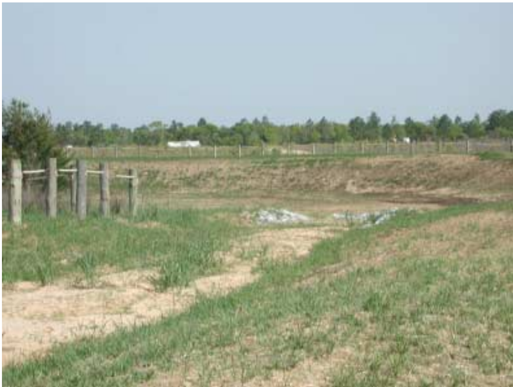
Retention Pond East of Sled Track Target Area
