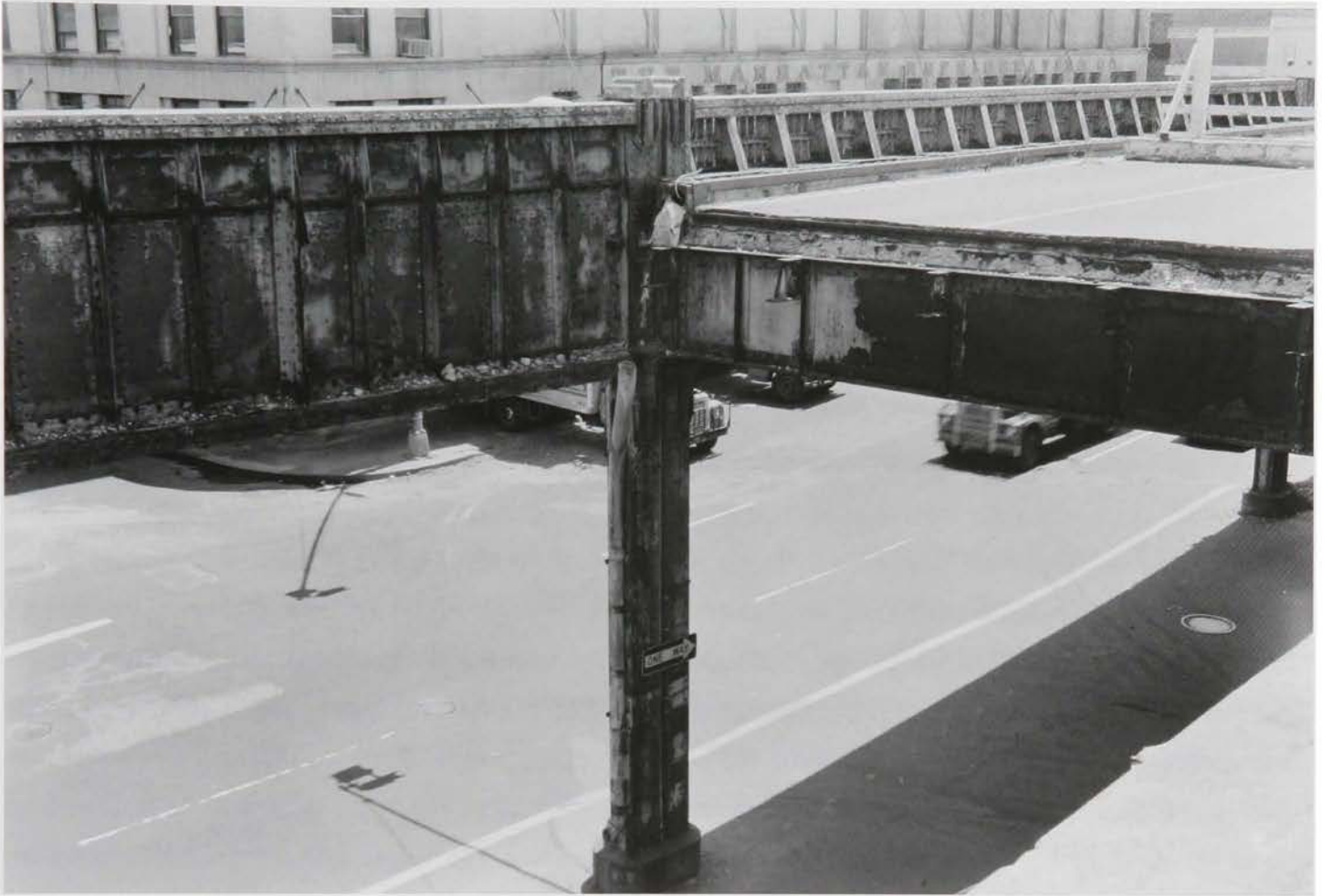
A collapsed section of the West Side Highway in Manhattan at 14th Street, circa 1974 [National Park Service]
