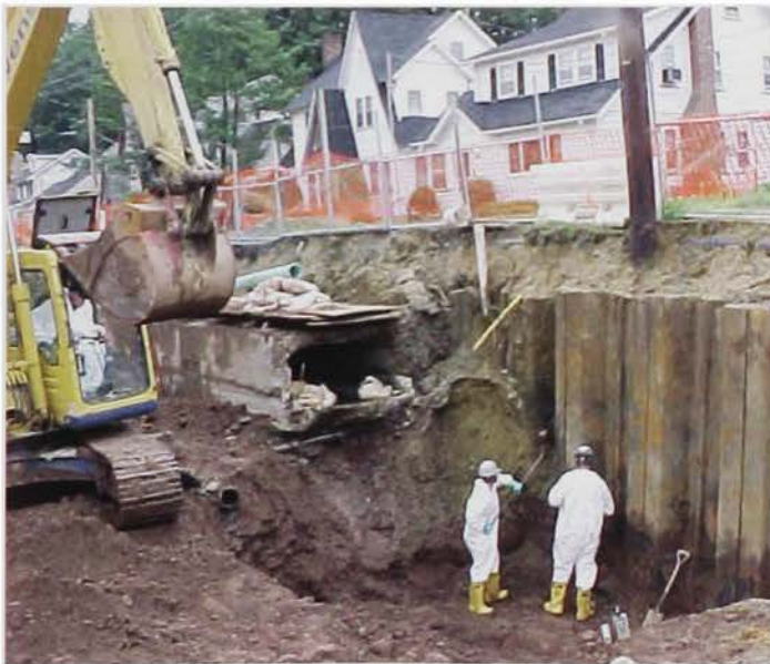
Workers wearing personal protective equipment dislodge contaminated soils from the sheetpile during remedial cleanup of a residential area in Montclair, New Jersey, circa 2000
