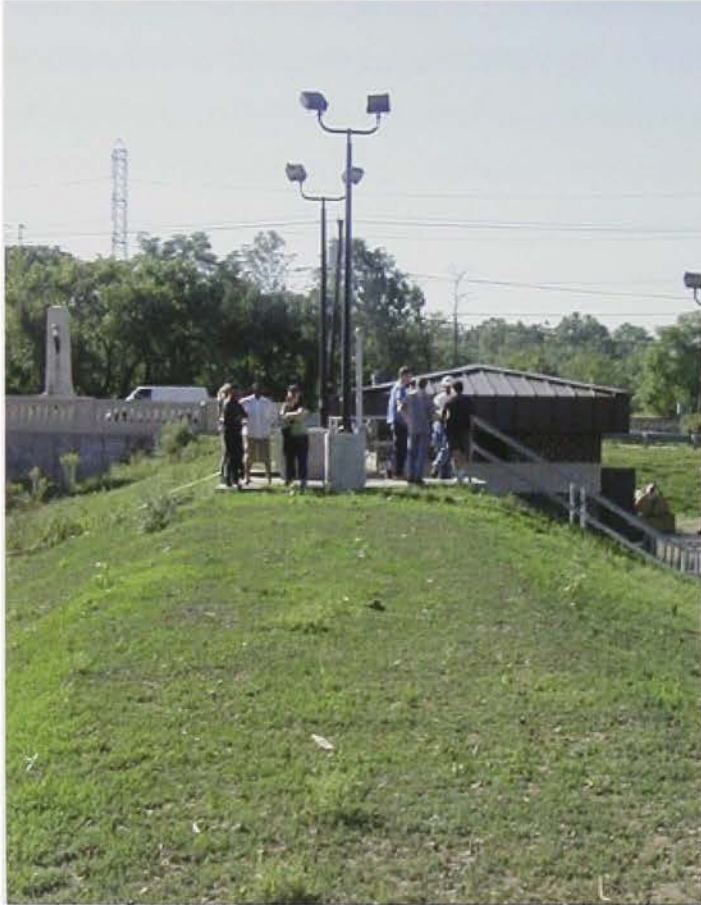
Pump station constructed in Bound Brook, New Jersey, for the Green Brook flood control project in 2005
