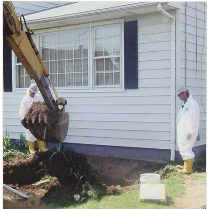
Removal of contaminated soil taking place adjacent to home at the Federal Creosote Superfund site in Manville, New Jersey, circa 2000
