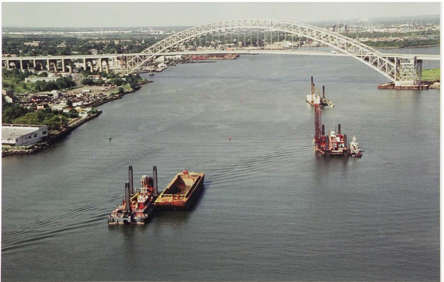
The dredge New York and accompanying scow (at left) and drilling rigs (at right) at work in the Kill van Kull near the Bayonne Bridge, circa 2005
