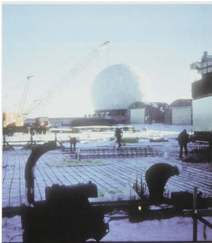
Construction in progress at Thule Air Base, Greenland
