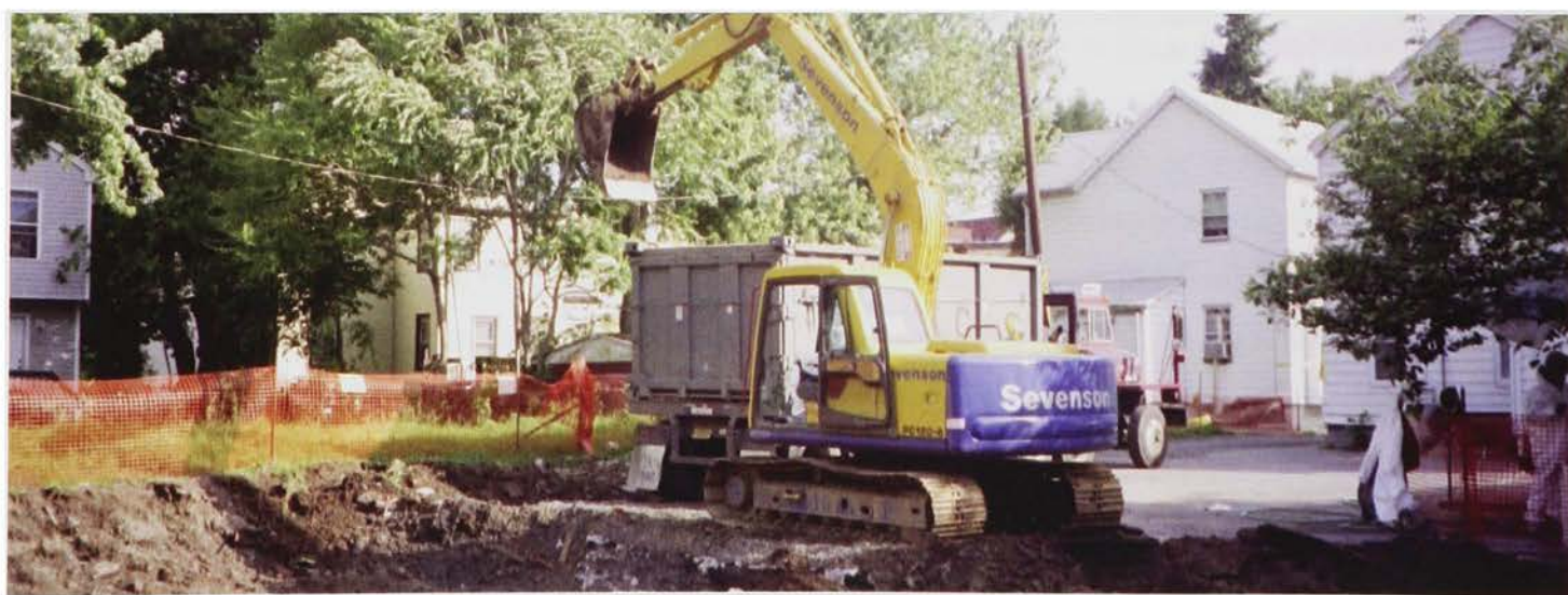
Workers wearing personal protective equipment excavate contaminated soil at the U.S. Radium Superfund site in West Orange, New Jersey, circa 1985
