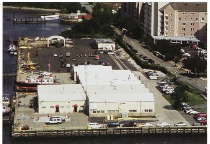
Caven Point Marine Terminal, Jersey City, New Jersey, where the New York District's floating plant is based
