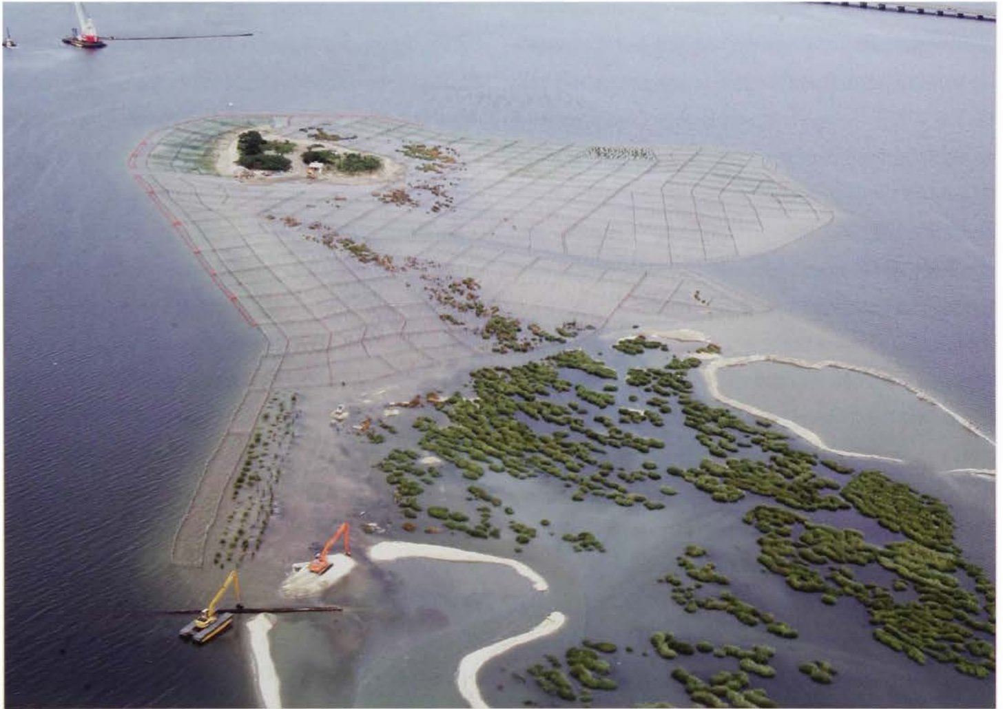
Replenishment of salt marsh with dredged sand at Elders Point Island, Jamaica Bay, New York in 2006
