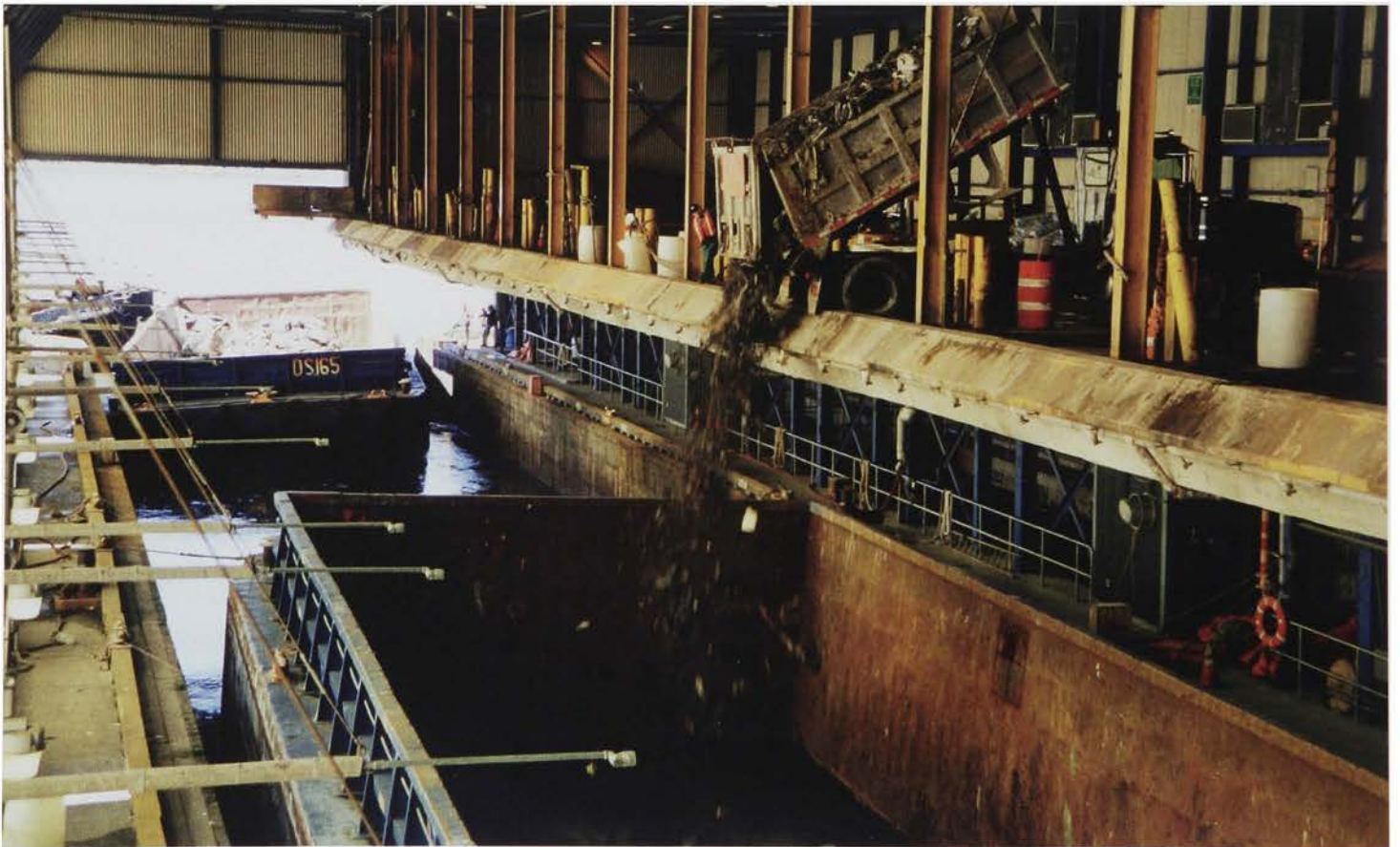
Barges being loaded with World Trade Center debris at Pier 6
