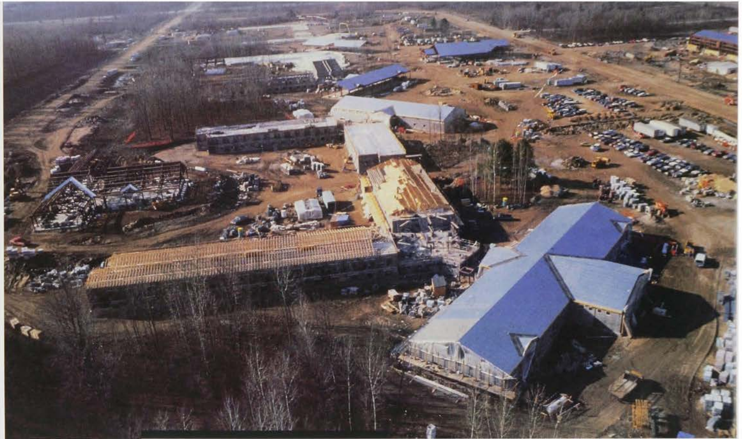
Fort Drum, New York, under construction, circa 1988
