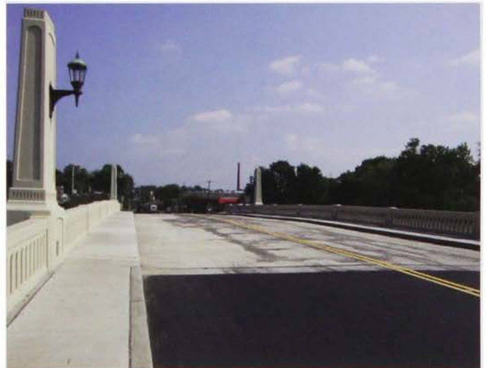
The new Lincoln Boulevard/East Main Street bridge in Bound Brook and Middlesex, New Jersey, rebuilt as part of the Green Brook flood control project, circa 2005
