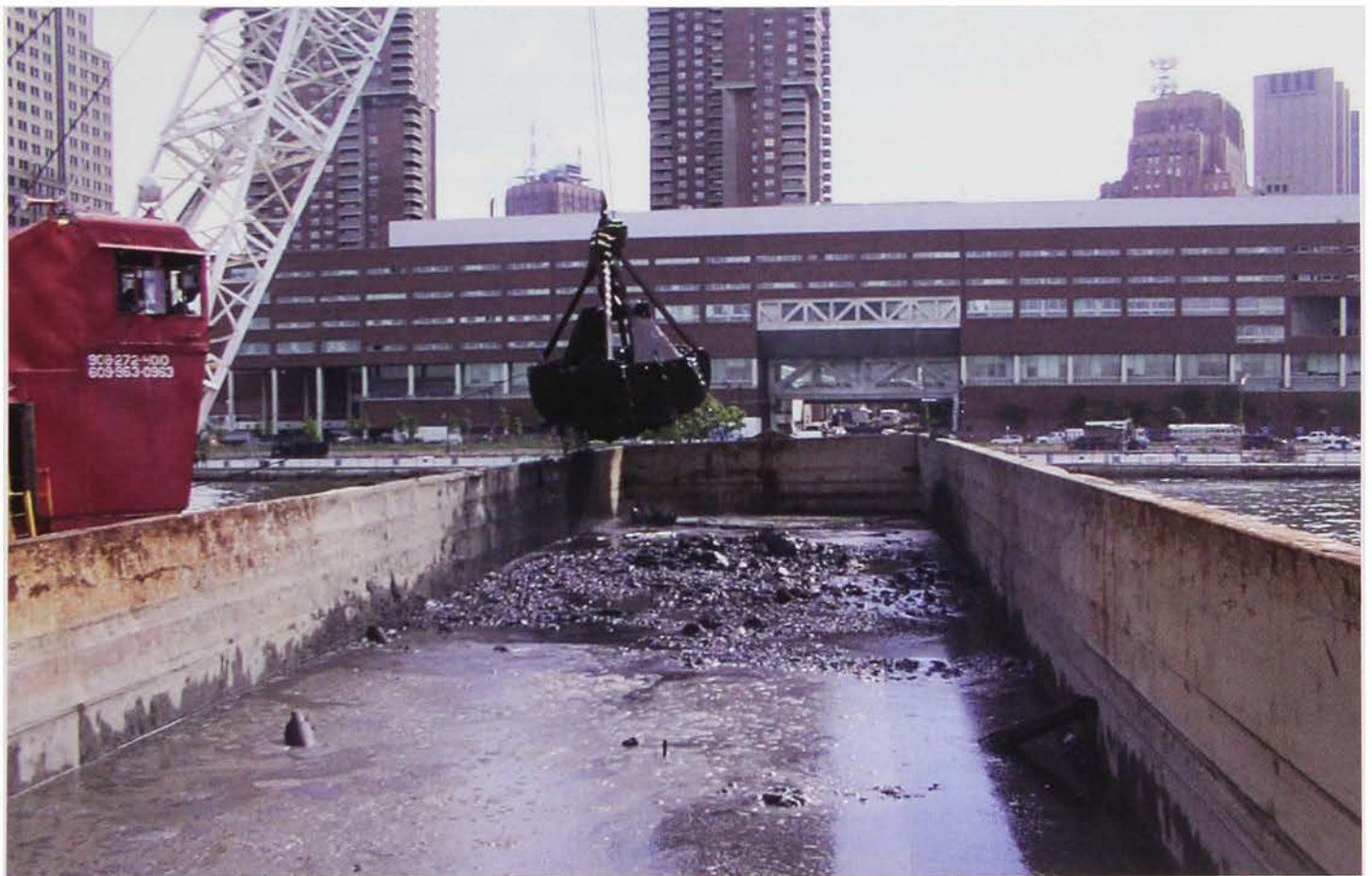
Clamshell dredge at work at Pier 25
