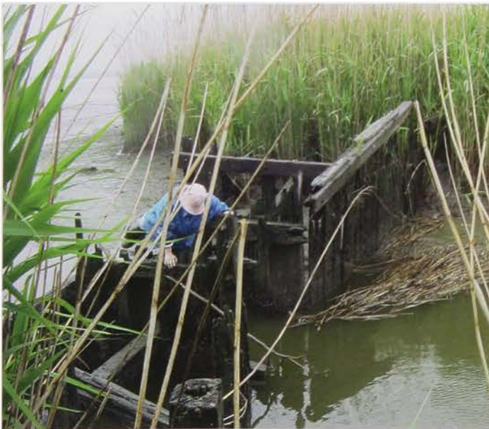
A New York District cultural resource specialist inspecting remains of a historic flood control structure in New Jersey's Hackensack Meadowlands
