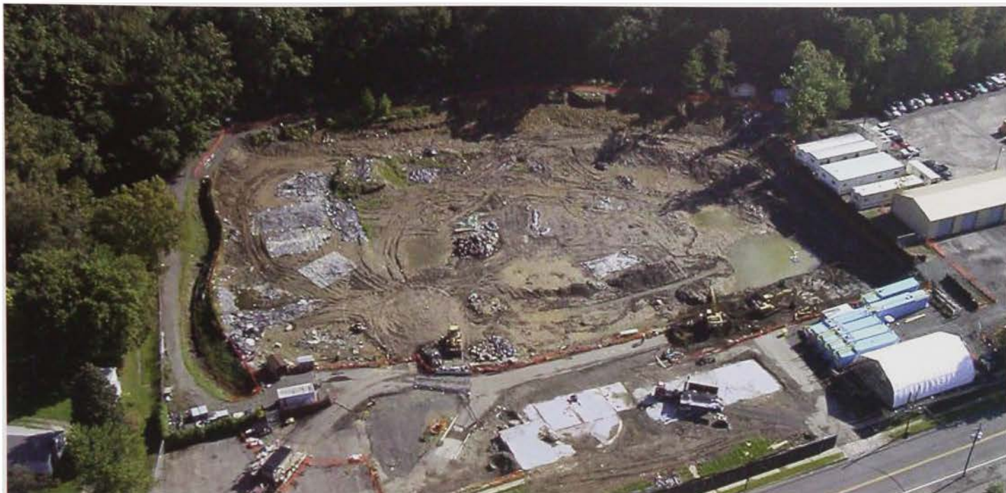
Cleanup under way at the Wayne Interim Storage Site in Passaic County, New Jersey, circa 2000
