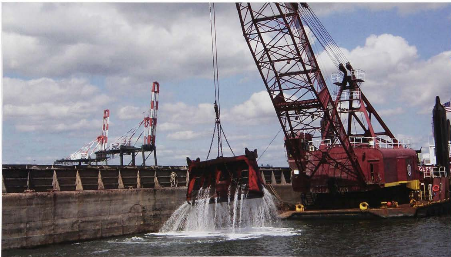
A clamshell dredge at work in the Arthur Kill in the late 1980s
