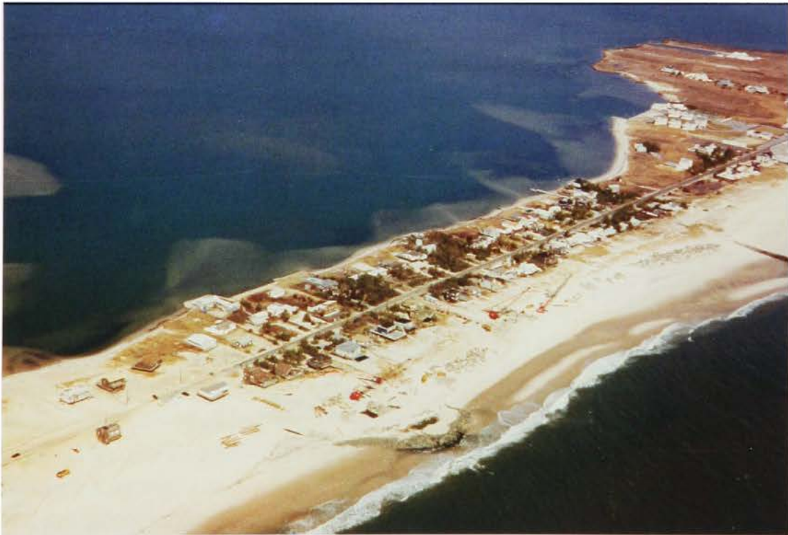
A section of the barrier beach in Westhampton, Long Island, New York
