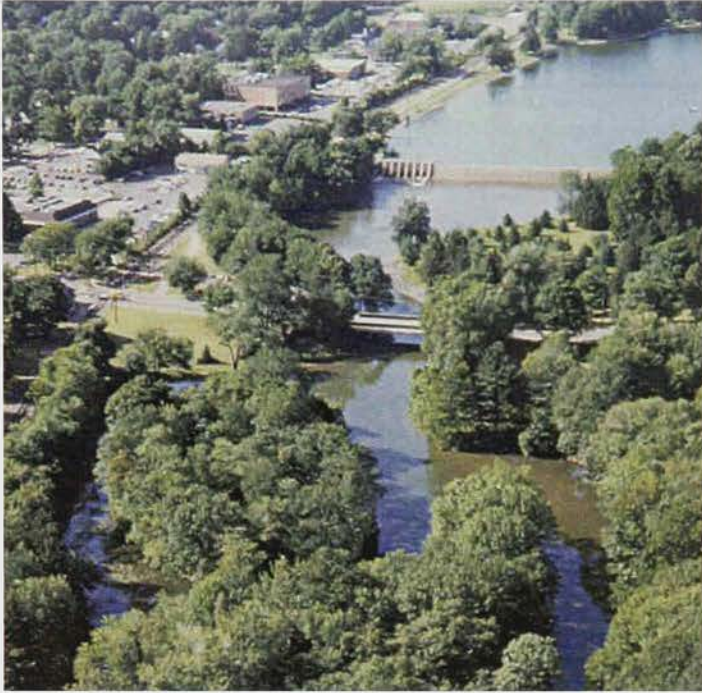
The Hackensack Water Company dam on the Hackensack River at Oradell, circa 1990 [New Jersey Meadowlands Commission]
