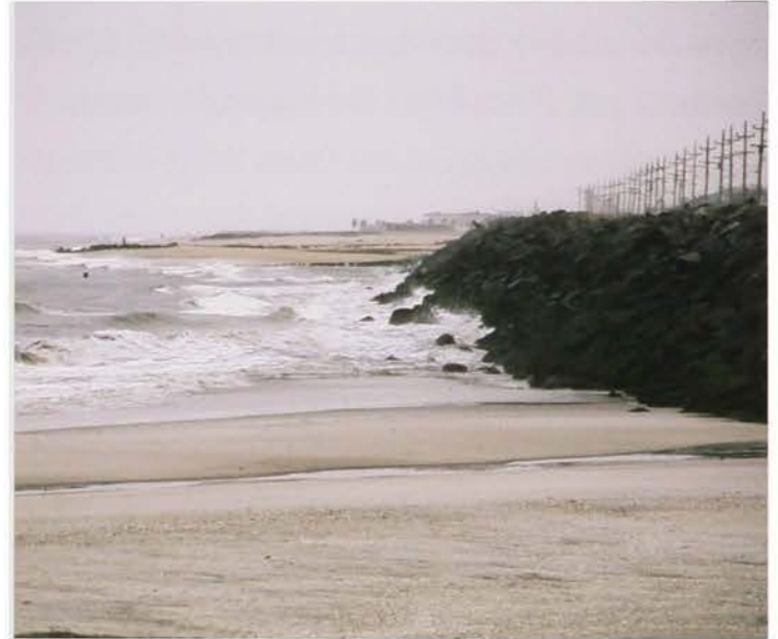
The Sea Bright seawall, Monmouth County, New Jersey, at low tide, circa 1980
