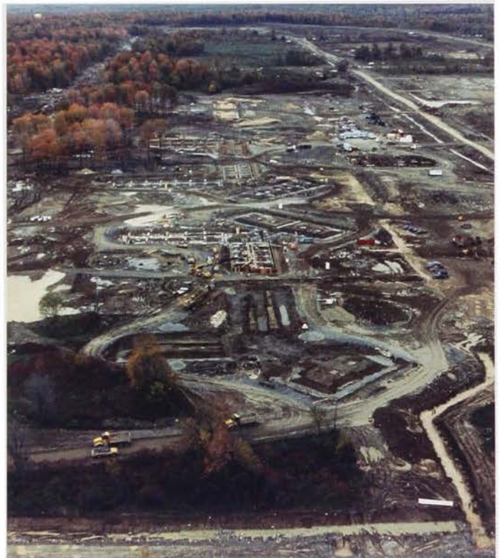
Site preparation in progress at Fort Drum in the late 1980s
