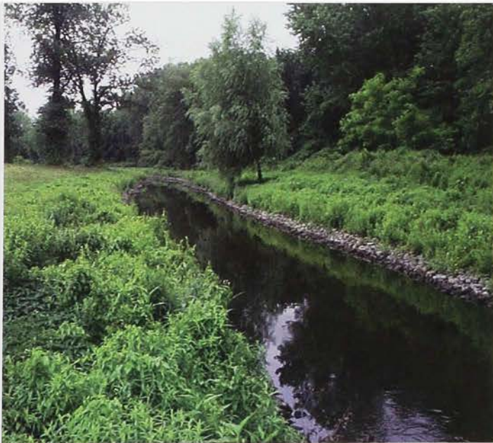
The channelized and rip-rapped Saw Mill River in Nepera Park, Yonkers, New York, circa 1998
