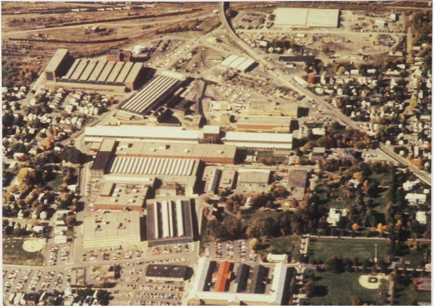
Aerial view of Watervliet Arsenal near Albany, New York, including the Benet Weapons Laboratory (red roof in foreground) and several weapons manufacturing facilities
