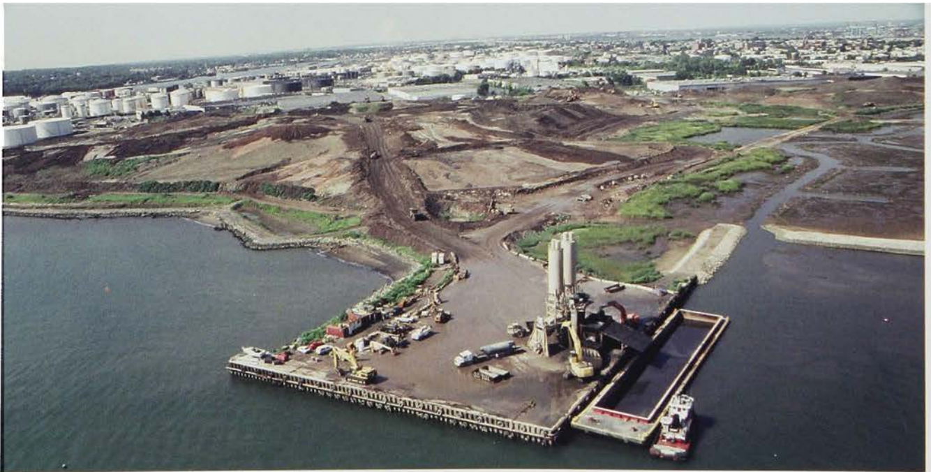
Dredged material being used to cap a brownfield in Bayonne, New Jersey, circa 2000
