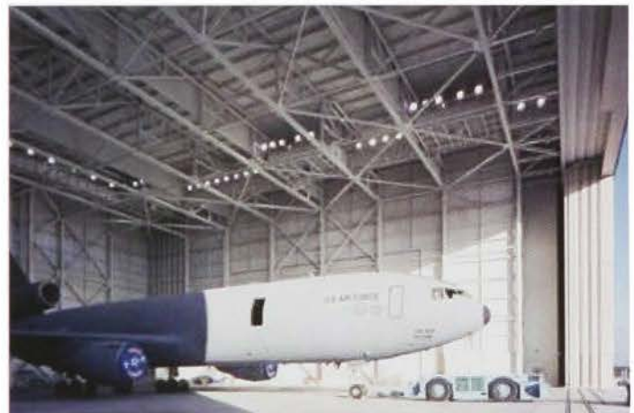
The interior of the KC-10 maintenance hangar at McGuire Air Force Base, Burlington County, New Jersey
