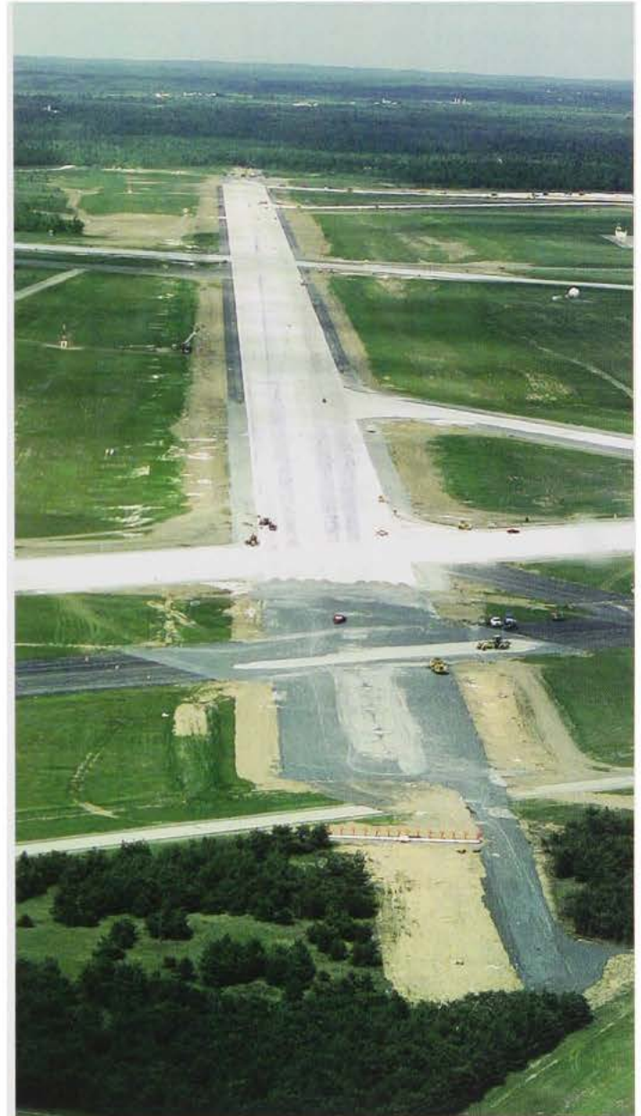
The airfield at Fort Drum, New York, under construction, circa 1991
