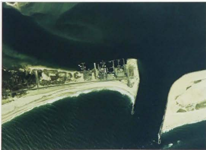
The strengthened and stabilized Shinnecock inlet, Long Island, New York, circa 2005
