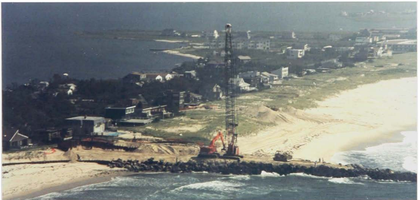
Scouring on the down-drift side of a groin along Westhampton Beach, Long Island, New York, circa 1996
