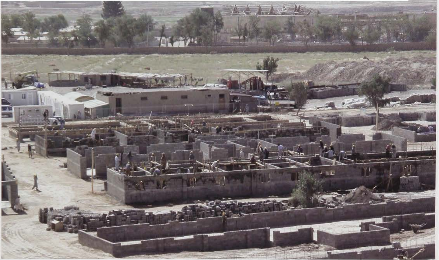
New construction in progress at the Afghan Army military base of Pol-e-Charki in 2003
