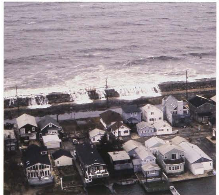
The Sea Bright seawall, Monmouth County, New Jersey, overtopped by Atlantic high tides, circa 1980
