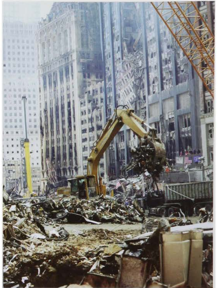
Debris removal at Ground Zero
