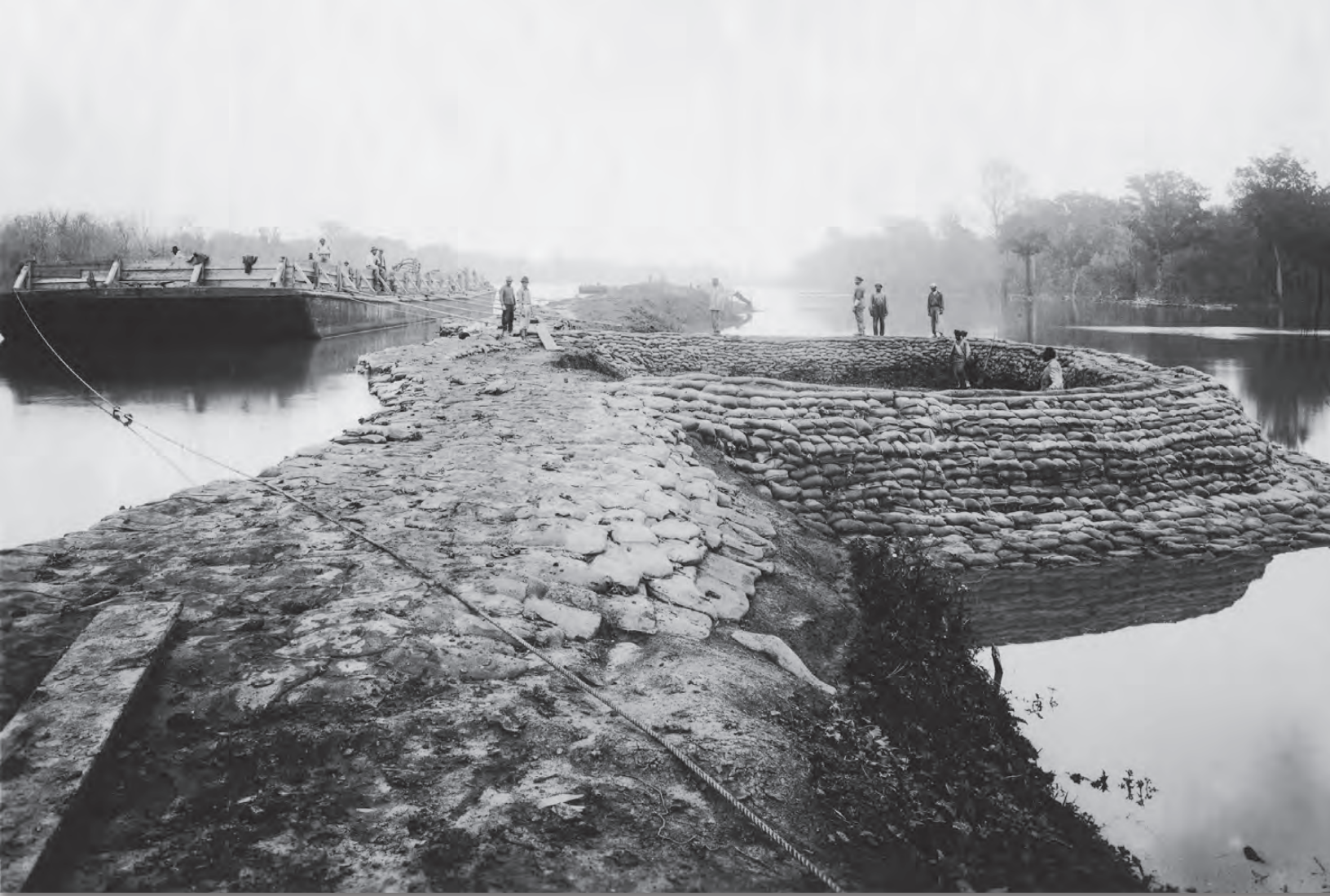
Workers added reinforcements to a threatened break in Ashbrook Dike on the Mississippi, 26 April 1922.
