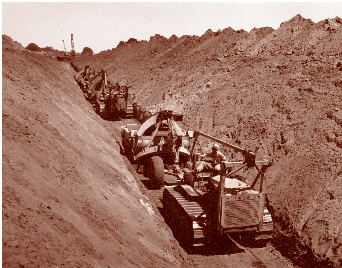
Engineers used heavy equipment to excavate Snead's Canal near Marianna, Florida, June 1948. The deepened canal drained floodwaters away from roads and buildings.
