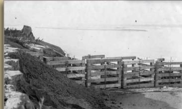
Concrete beam crib dike
