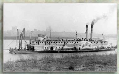
Captain Meriwether Lewis dredgeboat, capable of sucking and discharging 3,000 cubic yards of sediment an hour
