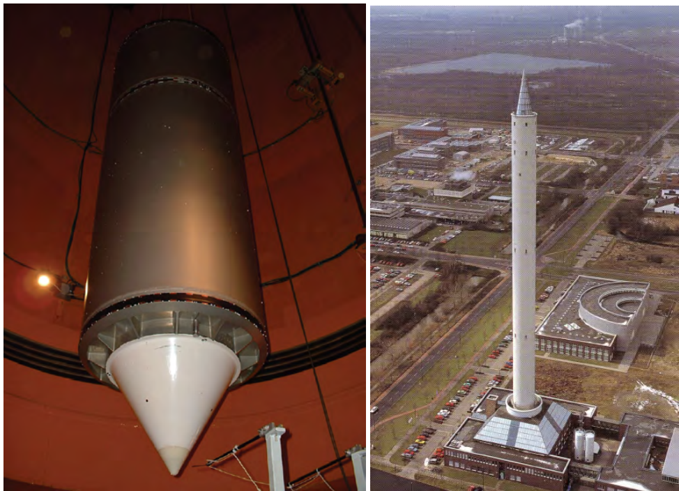
Fig.A.4 View of the drop capsule inside the ZARM Drop Tower, and aerial view of the tower.
