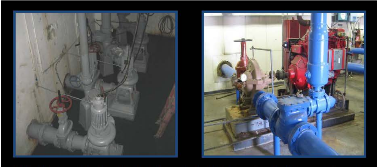
Figure 124. Examples of mechanical pumps associated with the oily waste and potable water systems on NSN.
