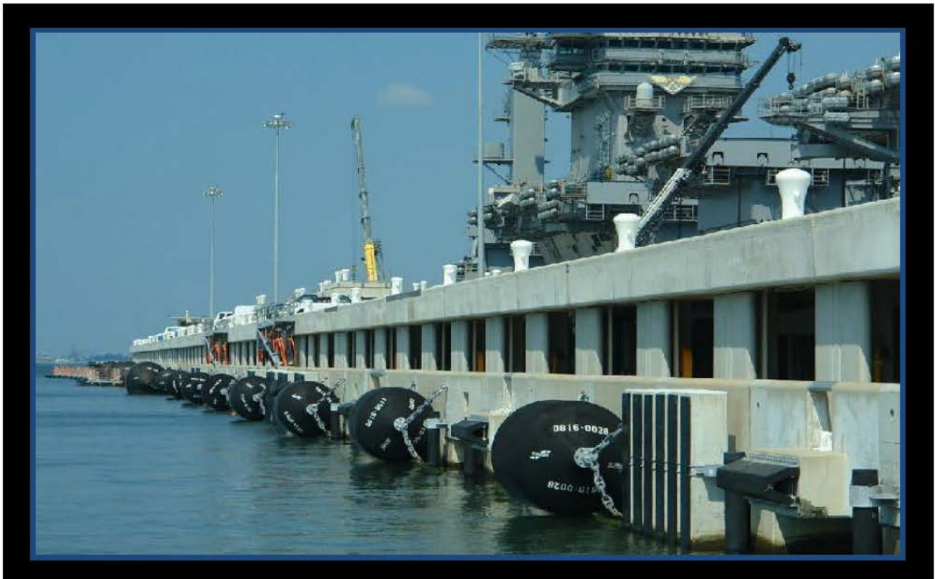
Figure 70. Pier 11 at NSN - an example of a shore-perpendicular structure in a heavily- altered coastal terrain with shore armoring, seawalls, and pavement (photo taken 23 August 2010).
