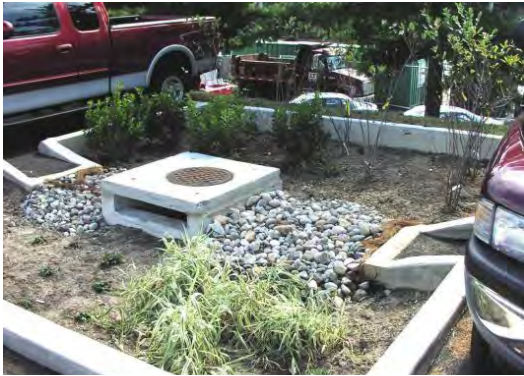
Figure 1 Bioretention Cell at Washington Navy Yard
