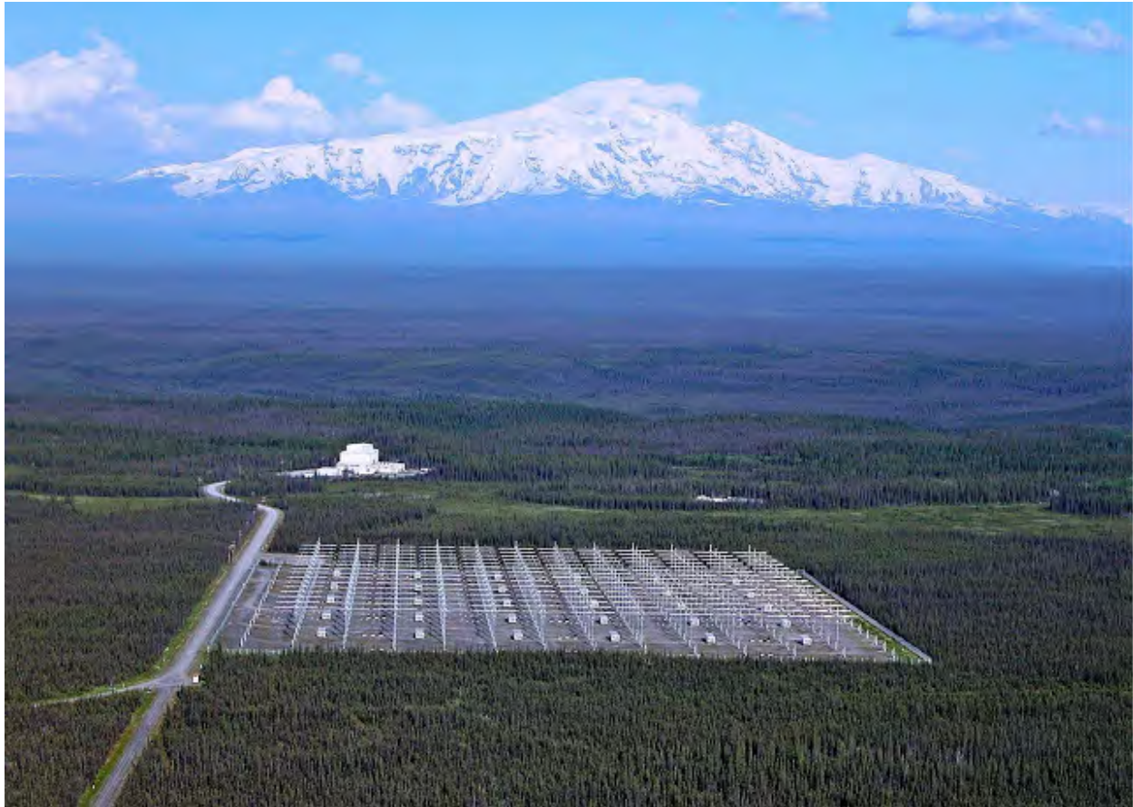
FIGURE S.1 Overhead photo of the High Frequency Active Auroral Research Program Gakona Facility. SOURCE: McCarrick, M., et. al., Marsh Creek LLC, “HAARP Facility Status,” presentation to the Committee on the Role of High-Power, High-Frequency-Band Transmitters in Advancing Ionospheric/Thermospheric Research: A Workshop, April 2013. Courtesy of M. McCarrick. Available at http://www.haarp.alaska.edu/haarp/photos.html .
