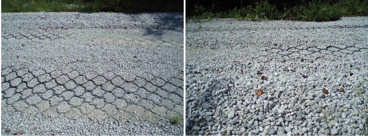
Figure A-9. Cross Section View of Road Deformation
