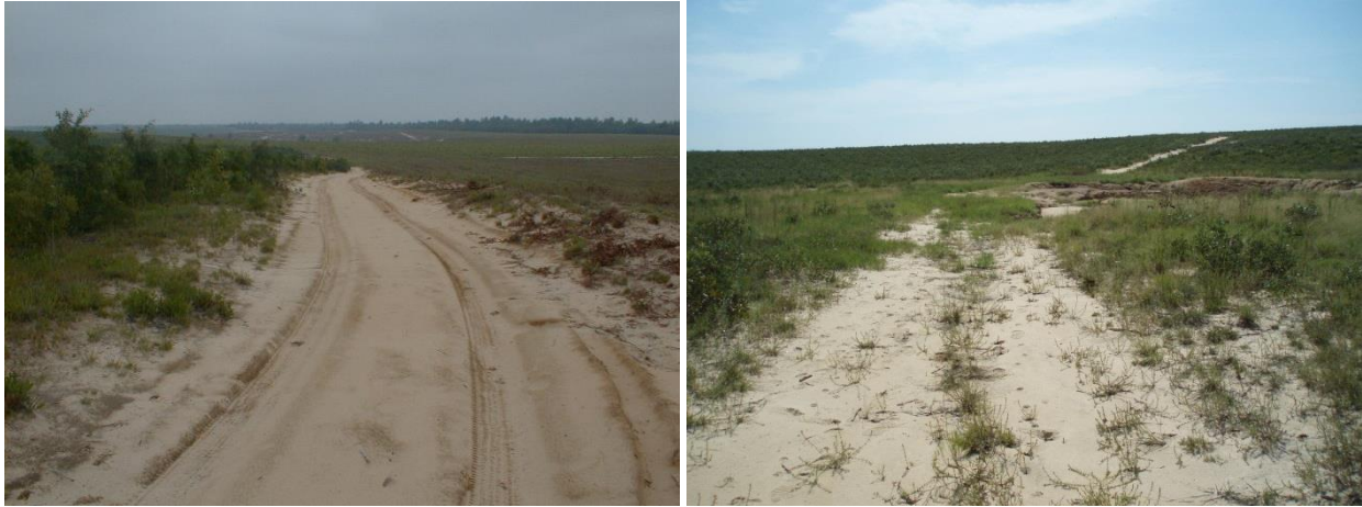
Figure A-5. TA C-74 Unpaved Road
