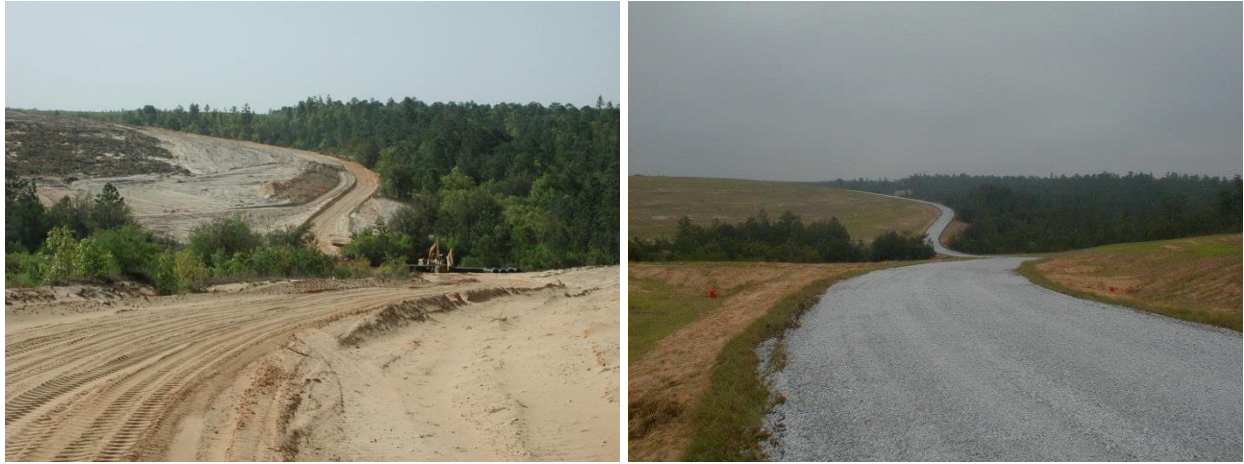
Figure A-6. TA C-74 Pre- and Post-Unpaved Road Reconstruction
