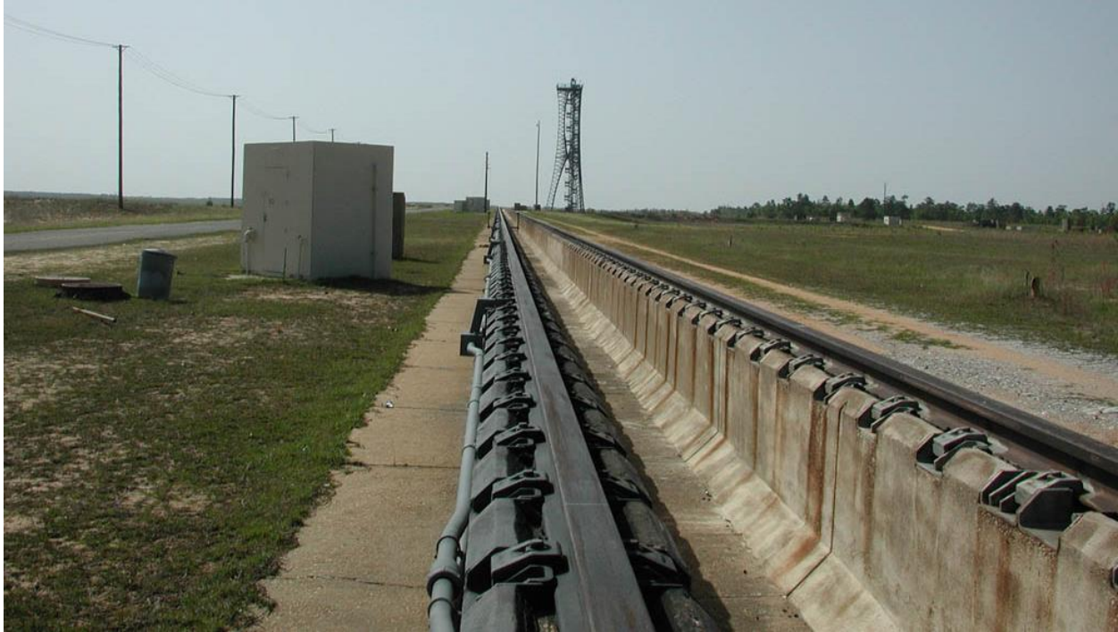
Figure A-2. TA C-74 KEMTF Sled Track and Observation Tower
