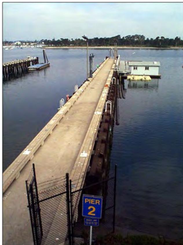
Figure 4-260. Small Craft Pier No.2, NAB Coronado. The pier is representative of 13 piers at NAB. The piers have fender systems for small craft, potable water service, and lighting.
