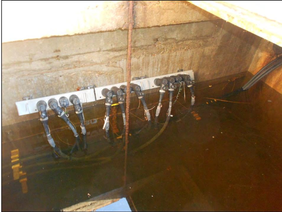
Figure 3-120. The photo shows a below-grade electrical vault partly full of water. A connection panel is visible above the water. The vault remains operational.
