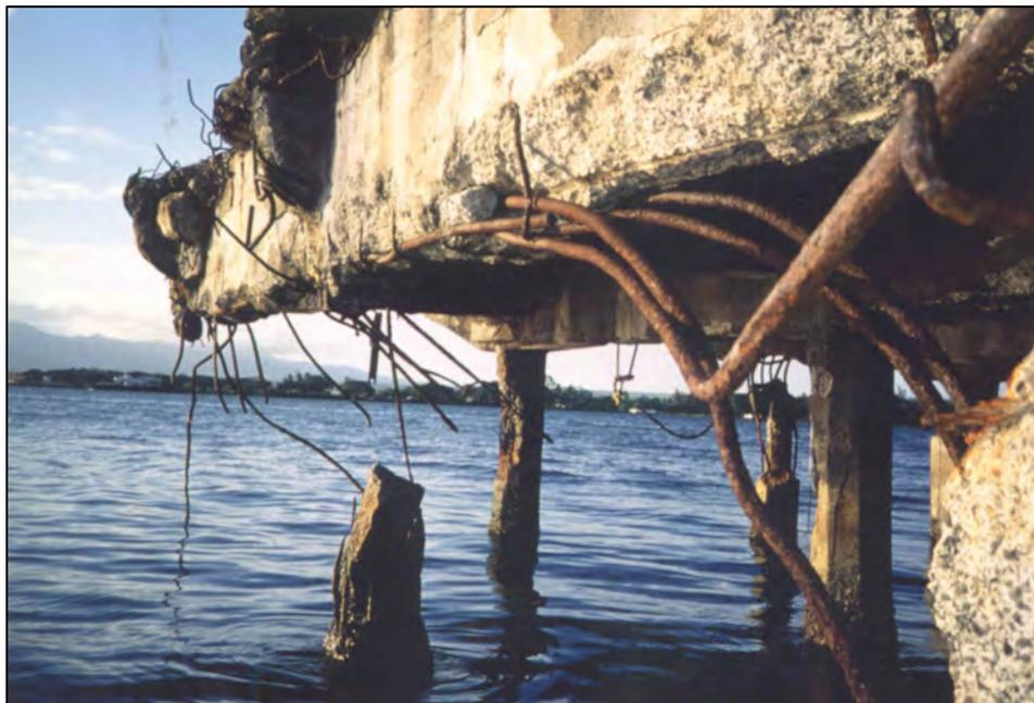
Figure 3-113. Waterfront structure that has excessive deterioration from chloride contamination and corrosion of the reinforcing steel (courtesy of Blaylock Willis and Associates).
