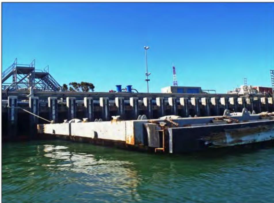
Figure 4-254. An aircraft carrier separator is a floating platform that provides clearance between the aircraft carrier and the wharf fender system, shown moored at Carrier Wharf Berth Kilo, NBC.
