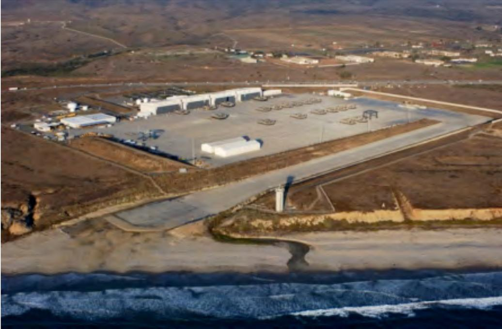
Figure 2-33. Oblique air photo of LCAC ramp taken 23 October 2004 and showing rough surface conditions at the end of the ramp, and a ditch from uncontrolled runoff (bottom center) in front of the tower (California Coastal Records Project Image 200407314; Copyright (C) 2002–2014 Kenneth & Gabrielle Adelman, California Coastal Records Project, [www.Californiacoastline.org](http://www.Californiacoastline.org)).
