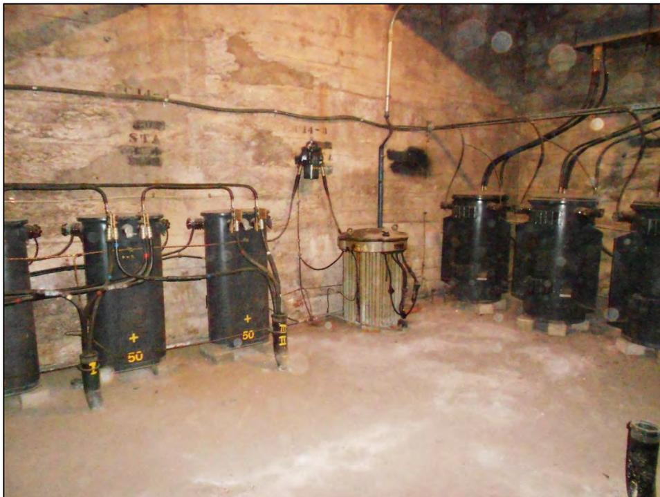
Figure 3-121. The photo shows an electrical vault with older equipment that has exposed connections and is susceptible to flood damage.
