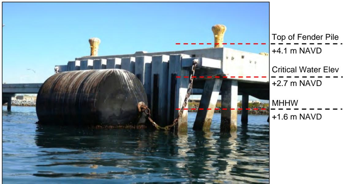
Figure 4-245. View of floating fender and concrete piles at Ammunition Pier Bravo, NBC. This system is vulnerable to “roll-over” with 0.5 m of SLR.
