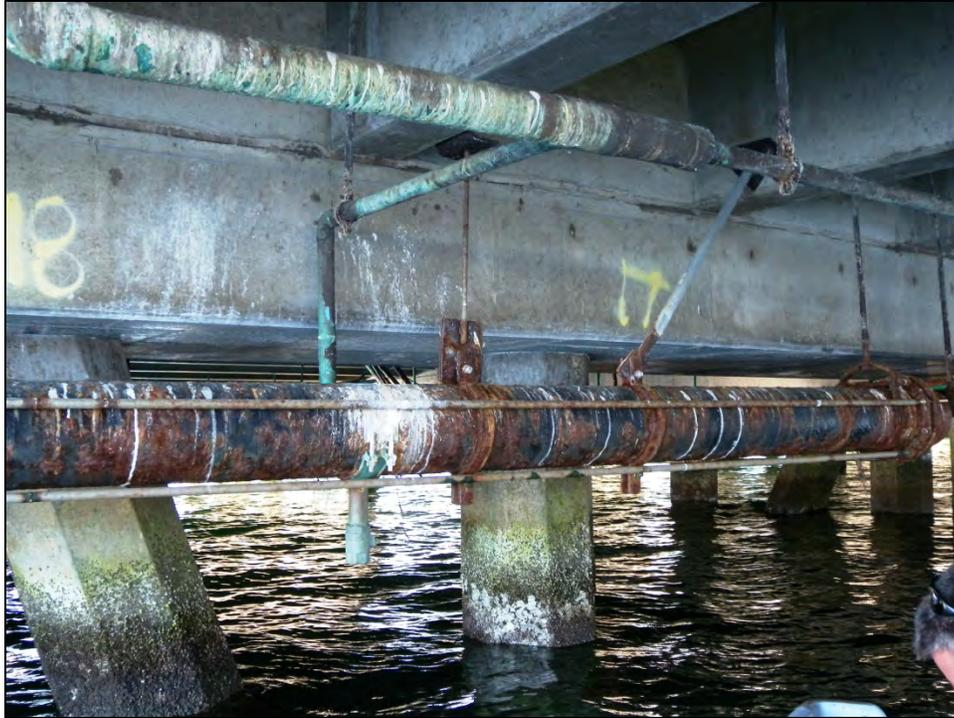
Figure 3-110. Pier with water pipe located below deck. The pipe and hangers may not be designed for wave and current loading.
