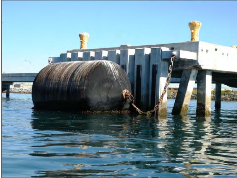
Figure 3-104. Typical pier fender system with floating fenders and concrete reaction piles at a close spacing for bearing.
