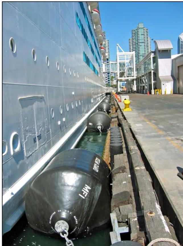
Figure 3-105. Foam filled fenders shown at high tide. With less than 1.0 m of SLR, "roll-over" could occur.
