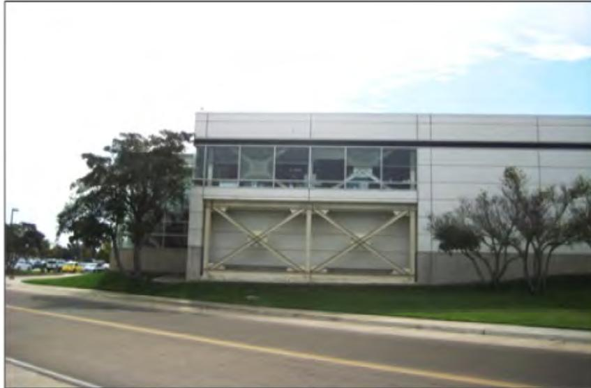
Figure 4-236. Naval Base Coronado with the Helicopter Training Facility as seen from Moffett Road. The exterior surface (lawn) berms up towards the building to lessen the impact of the wall elevation. The interior finish floor is approximately 30-in. below adjacent exterior grade.
