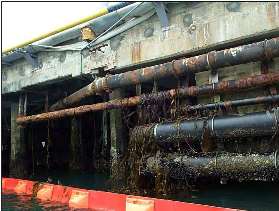
Figure 3-109. Pier with utility pipes located below deck in the tidal zone. The pipes are submerged during high tides and collect kelp and other debris.
