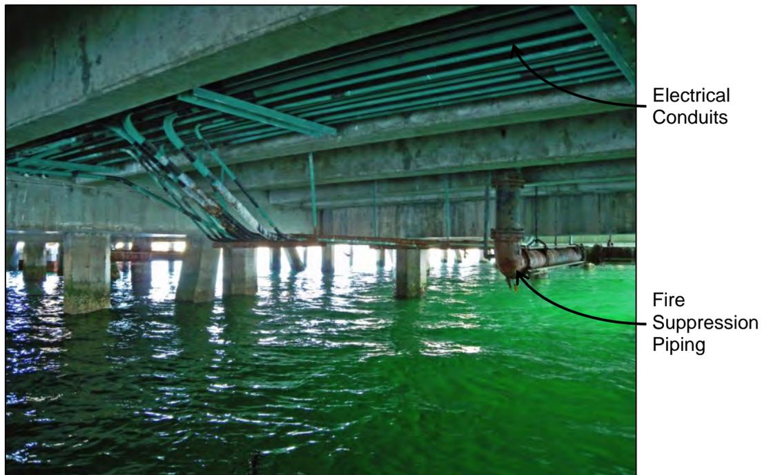
Figure 4-246. The fire suppression piping and electrical conduits at Ammunition Pier Bravo are located below the pier deck.
