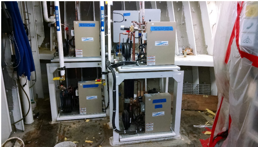
Refrigeration Contractor aboard pressure testing piping between ships refer plants and compressors in BT space. Science Refer piping pressure testing scheduled for tomorrow.
