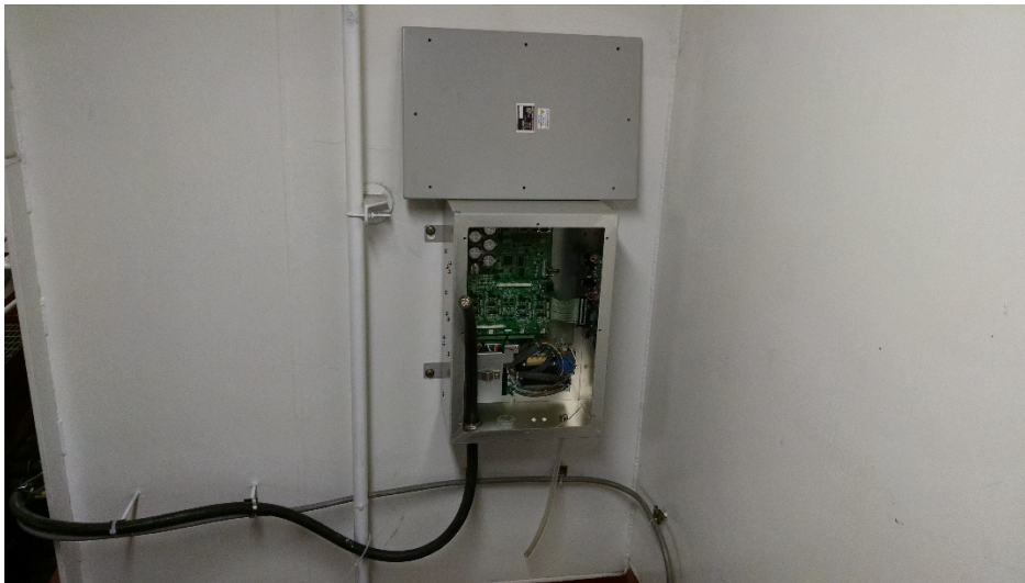
Upgraded cable installed to connection box in transducer room for bridge speed log. Replacing this cable seemed to remedy speed log issues on Armstrong.
