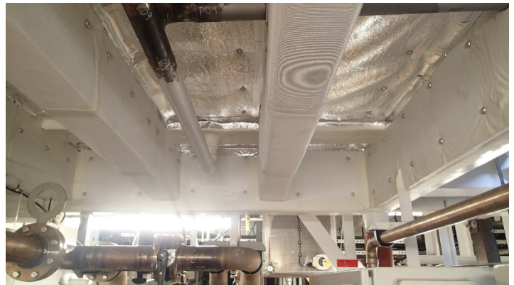
Engine Room Overhead Aft – Quad-Zero and Mylar Sheathing
