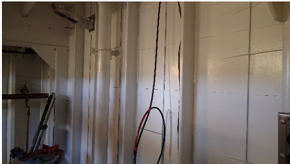
Traction Winch Rm fwd bulkhead tiles
