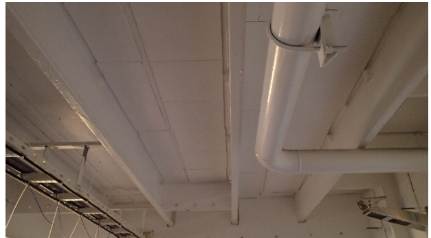
Traction Winch Rm Overhead tiles.
