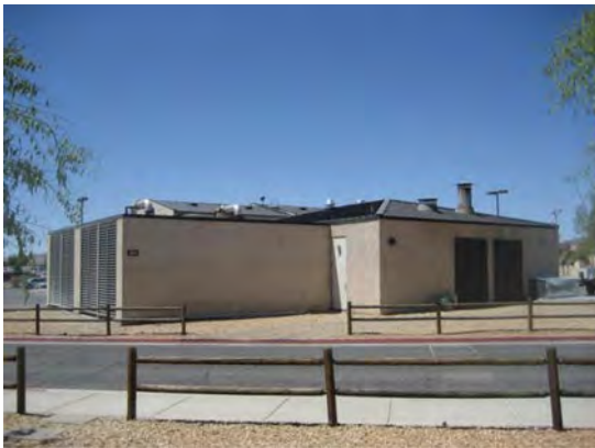
Central Cooling Plant, Bldg. 263 (7th St. off Barstow Rd.)
