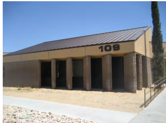
Central Cooling Plant, Bldg. 109 (Langford Lake Rd. off 'B' Ave.) (Mechanical room is at the rear of the building)
