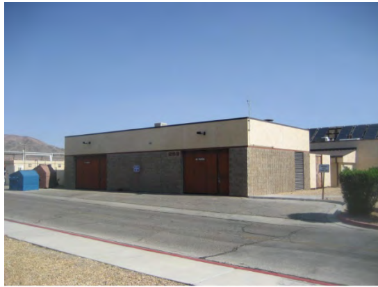
Central Cooling Plant, Bldg. 253 (4th St. off 'B' Ave.) (Chiller mechanical room is on the left side of the building)
