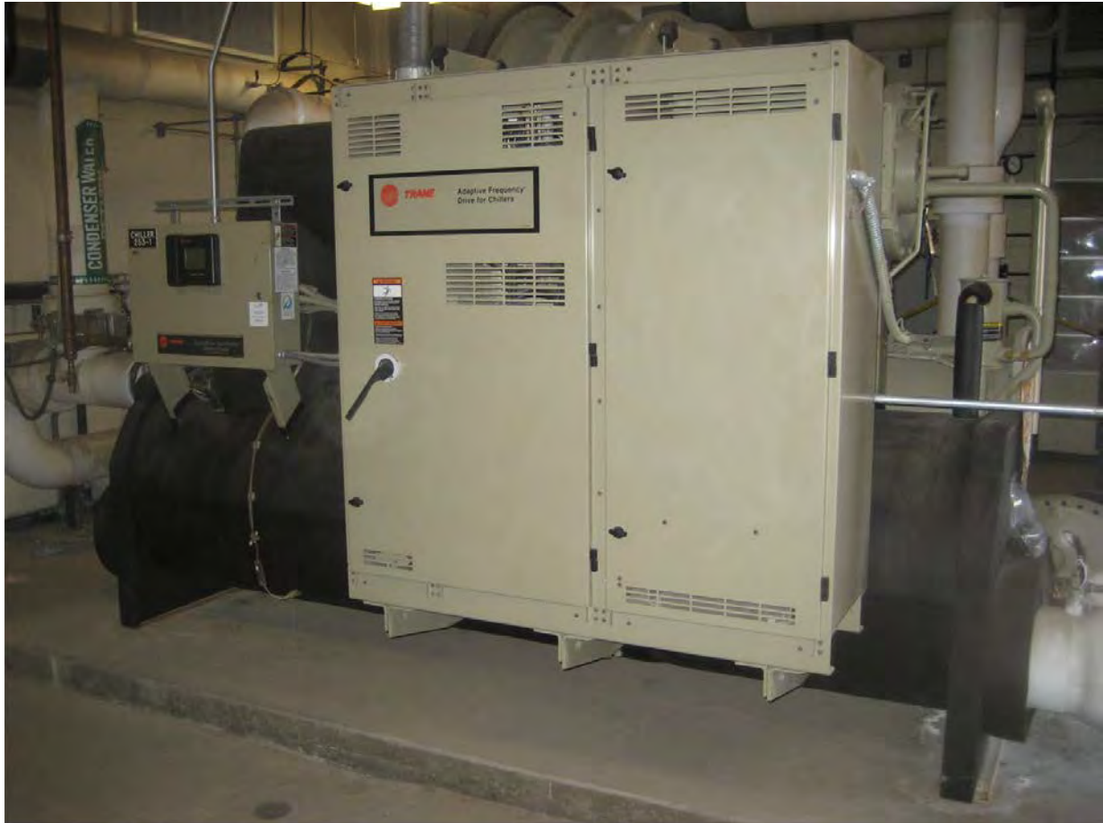
Figure 8. Chiller: Building 253 Central Cooling Plant
