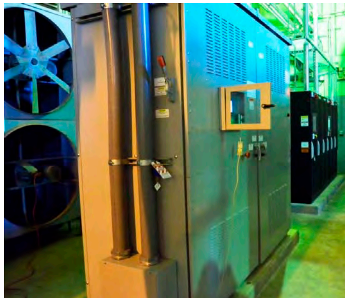
Figure 7. 500kW storage inverter.
