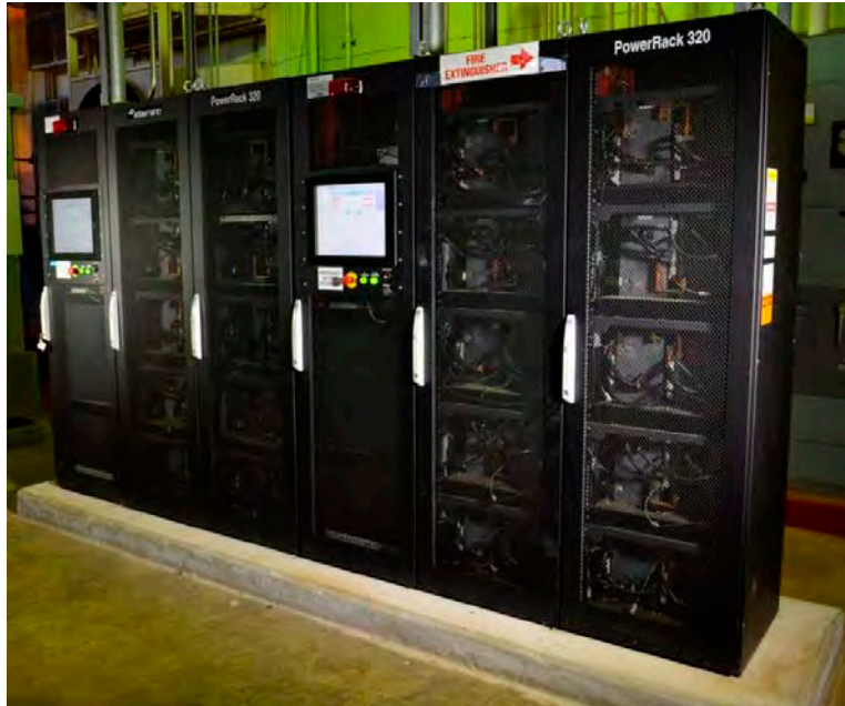
Figure 6. 400kW power optimized storage battery.
