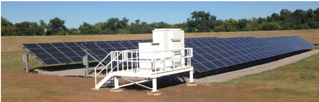
Figure 5. 86kW PV array and PV inverter.
