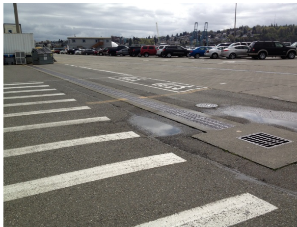
Figure 1-2. Drain for Untreated Runoff
