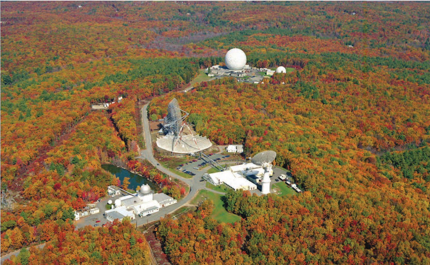
Lincoln Space Surveillance Complex, Westford, Massachusetts
