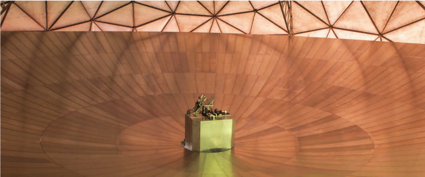
The Haystack Ultrawideband Satellite Imaging Radar (HUSIR) 37-meter-diameter primary reflector surface achieved its final precision alignment goal, allowing final dual-band (X and W) integration and testing to proceed in preparation for transitioning HUSIR to operational use in the U.S. Space Surveillance Network.
