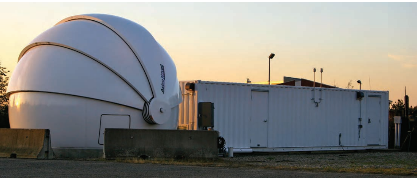
The closed-up clamshell dome for LLCD's ground terminal sits adjacent to the converted shipping container that houses all the control and modem electronics, laser transmitters, and the unique receiver, as well as the control room.
