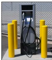
Eaton AC charging station - LAAFB (Supports AC charging)
