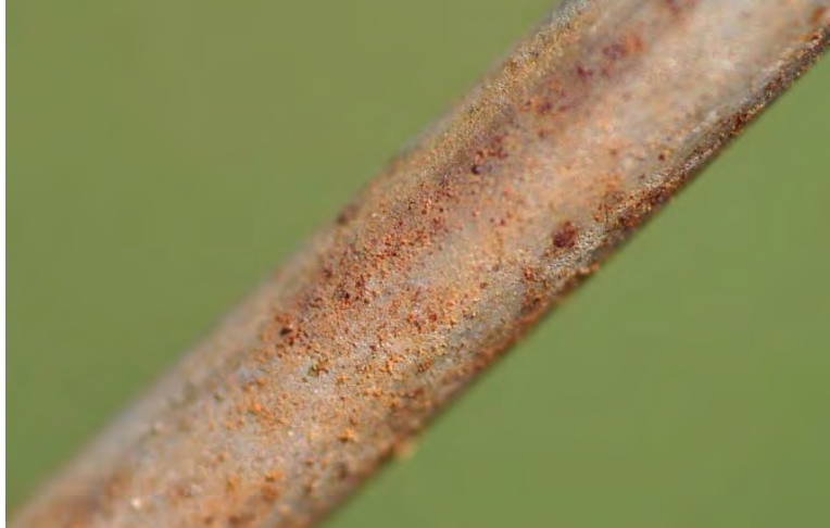
Figure B133. Stainless Steel Wire Fencing
