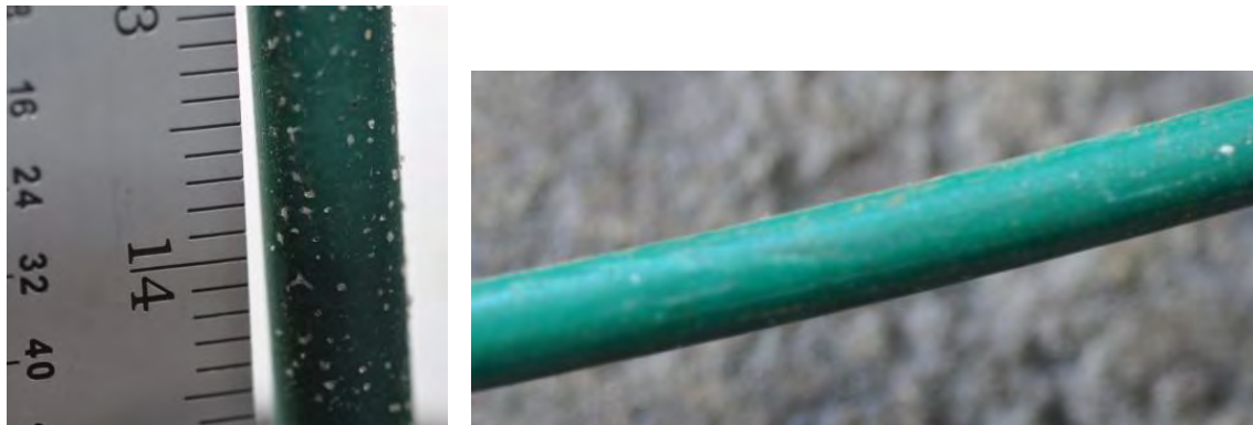
Figure 25. Fuse bonded PVC coated wire coupon at FRF (left) and KTA (right) after 12 months of exposure.
