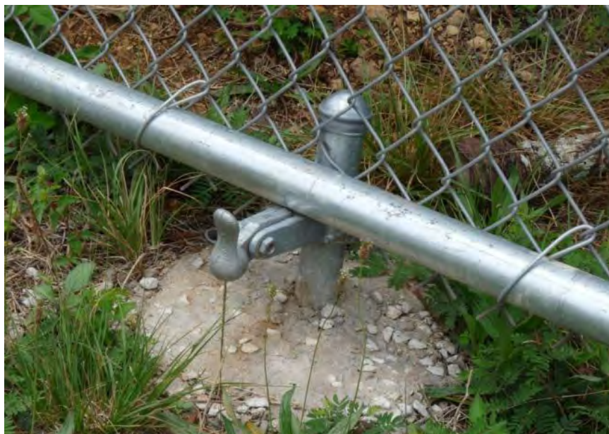
Figure 6. Position-locking hardware for vehicle gates.
