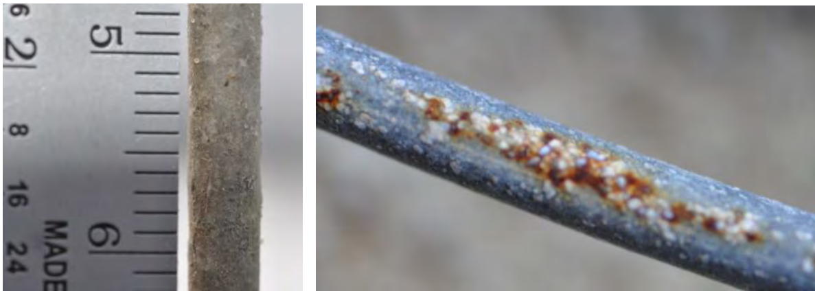
Figure 23. Standard galvanized steel wire coupon at FRF (left) and KTA (right) after 12 months of exposure.
