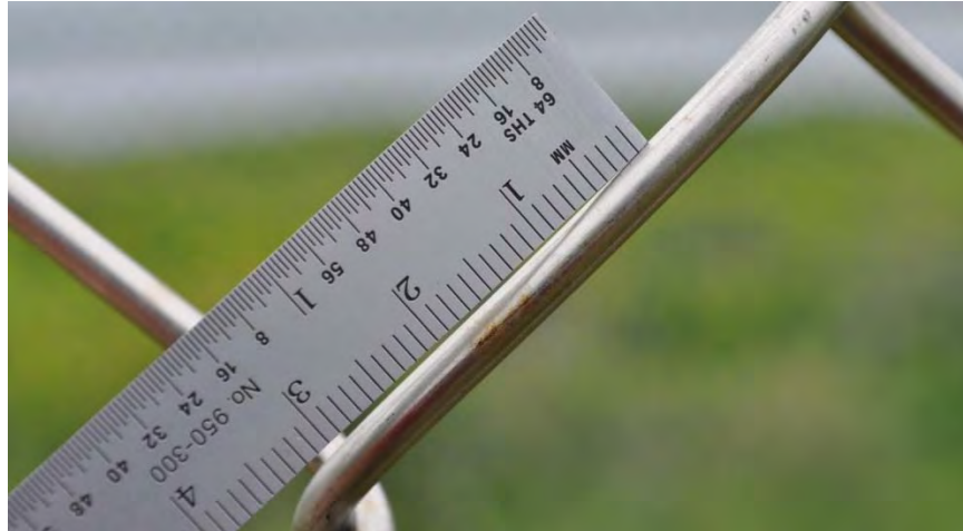
Figure B18. Stainless Steel Wire Fencing
