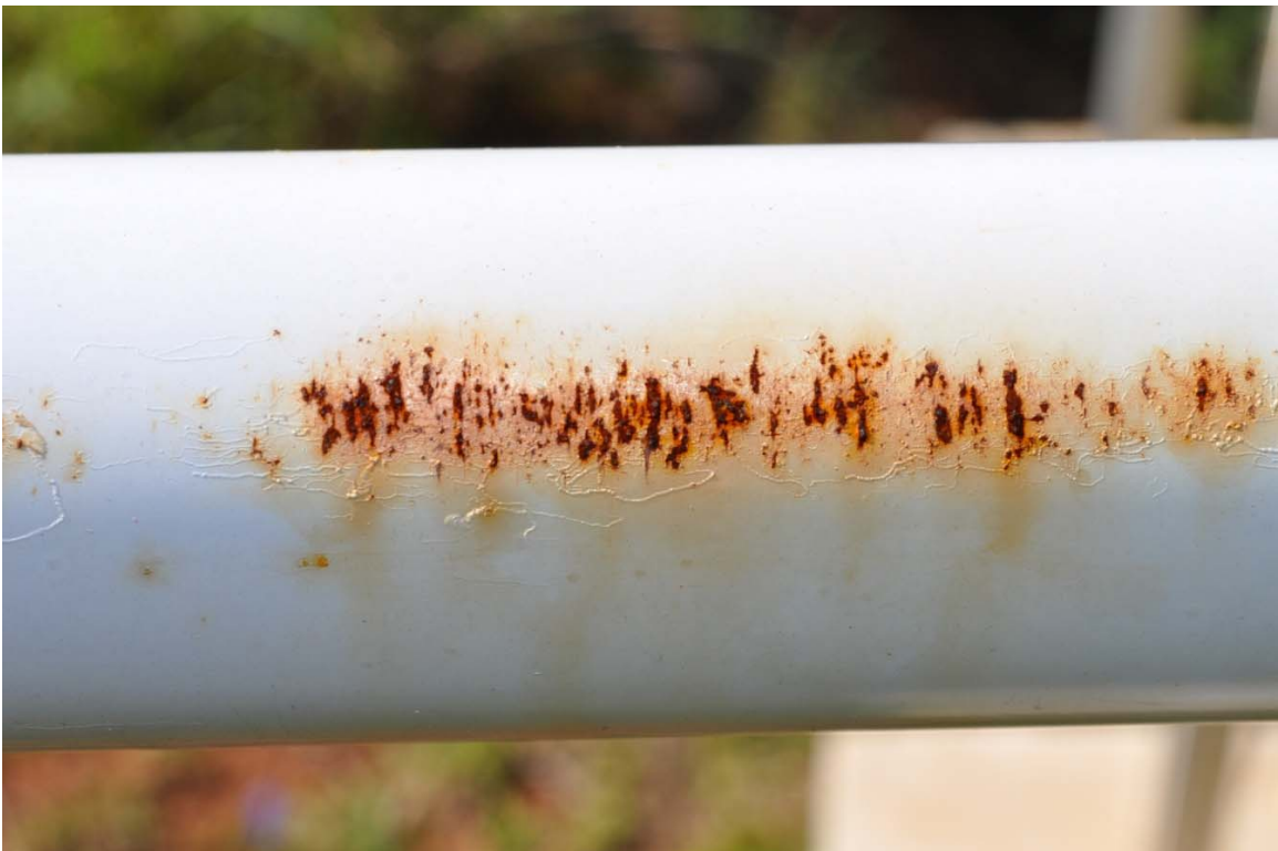
Figure B120. Coated Steel Railing
