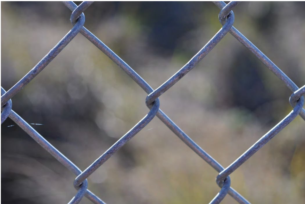
Figure A10. Galvanized steel after 6 months exposure.
