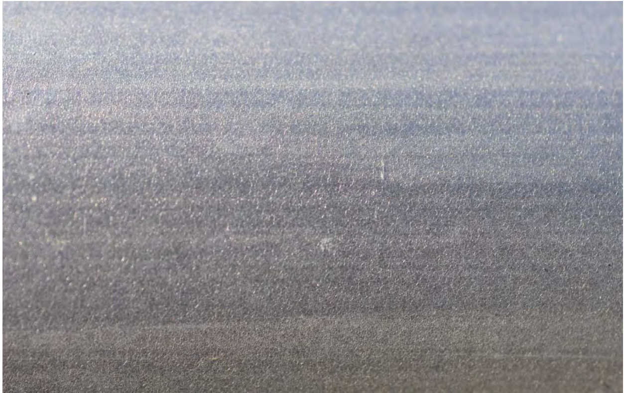
Figure B123. Aluminum Railing Coupon
