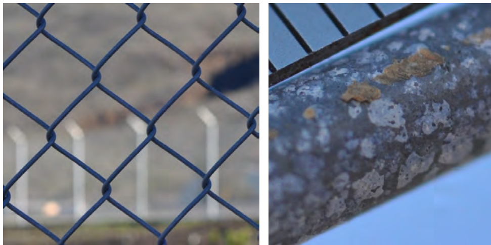
Figure A16. Galvan showing localized corrosion on 10% of its total surface after 12 months exposure.
