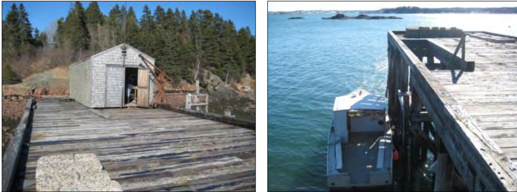
Figure 3. Treat Island weathering station wharf, view toward location of exposure racks and weather station (left) and end of wharf showing access stairway (right).
