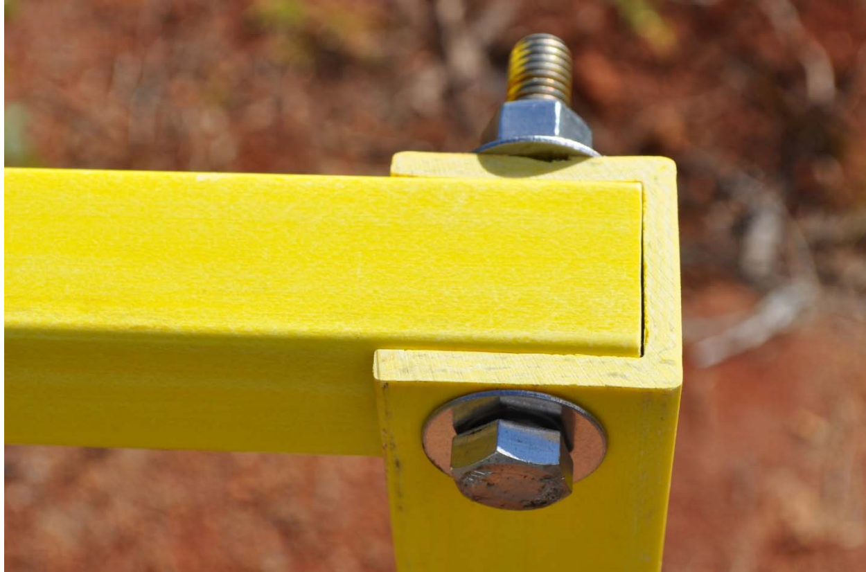
Figure B78. Fabricated FRP Railing
