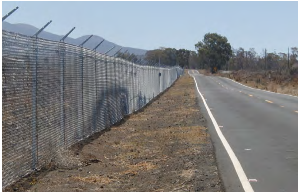
Figure A2. Galfan fence at south end BAA perimeter adjacent to Old Saddle Road.
