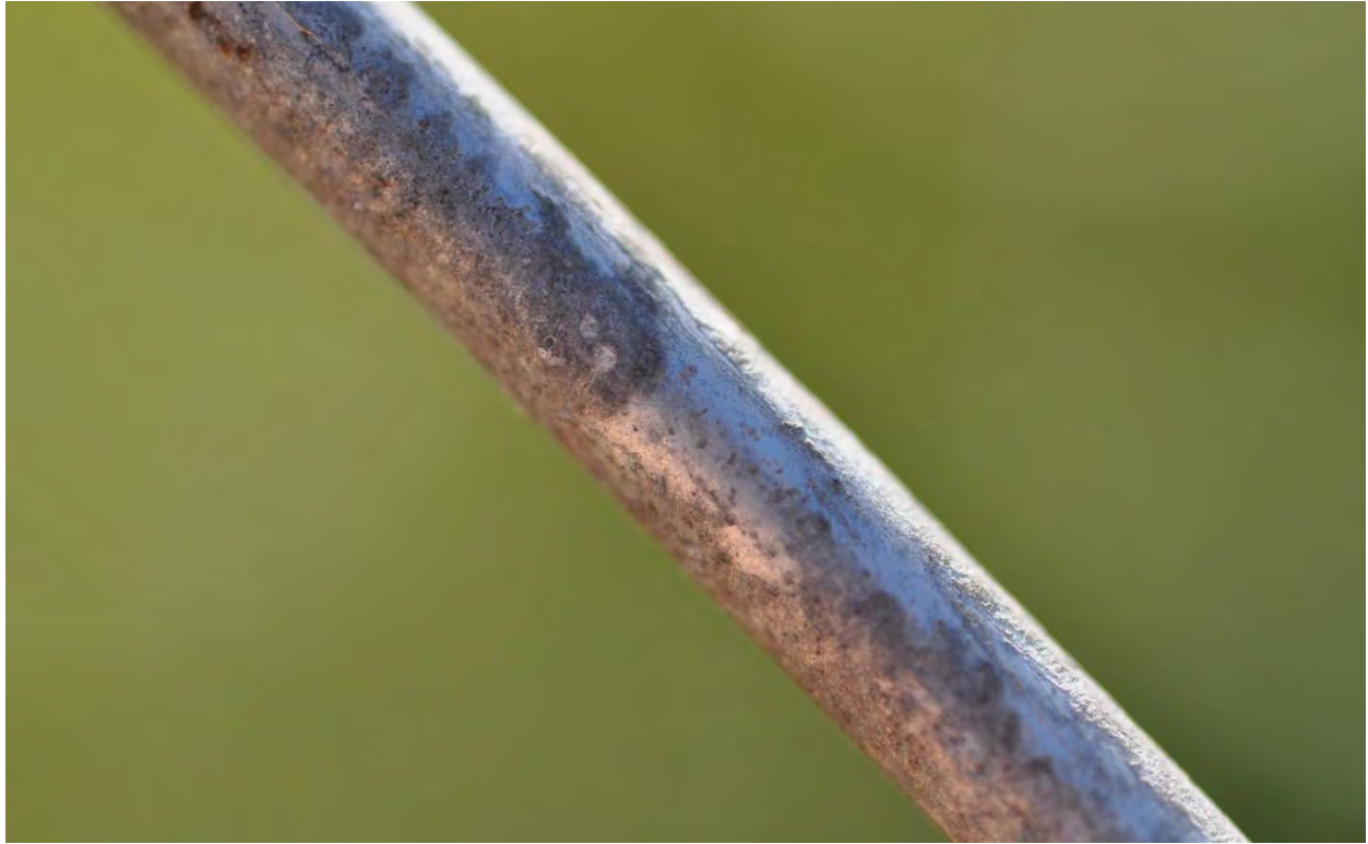
Figure B127. Aluminized Steel Wire Fencing
