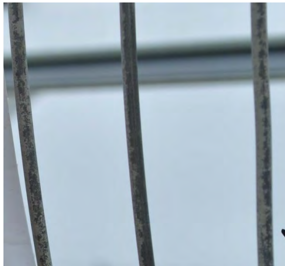
Figure B13. Aluminized Steel Wire Coupon
