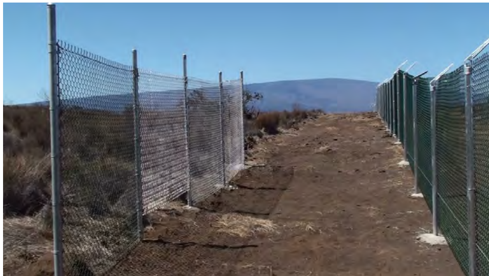
Figure A3. Fuse-bonded PVC fencing at west BAA perimeter from Old Saddle Road to New Saddle Road (right) and four test sections of control materials (left).
