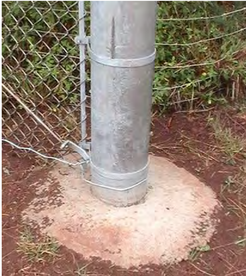
Figure 5. Fencing pole anchored in concrete.
