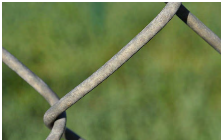
Figure B41. Galvan Wire Fencing
