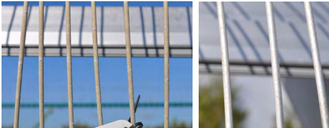
Figure 19. Aluminum wire coupon at FRF (left) and KTA (right) after 6 months of exposure.
