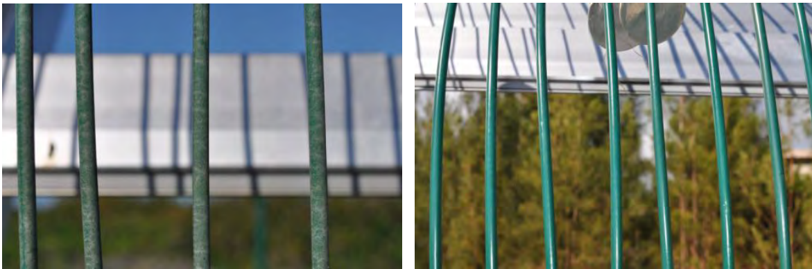
Figure 18. Standard PVC coated galvanized wire coupon at FRF (left) and KTA (right) after 6 months of exposure.
