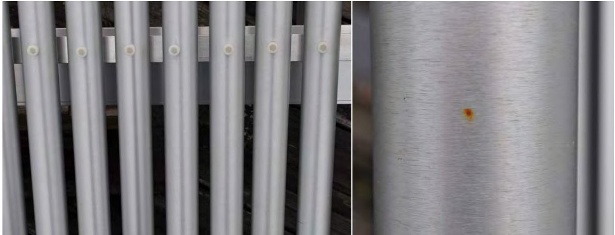
Figure B152. Aluminum Railing Coupon
