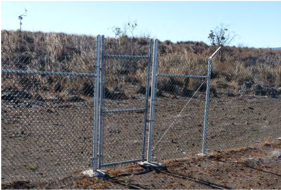
Figure A4. Personnel gate with three rows of barbed wire and locking hardware.
