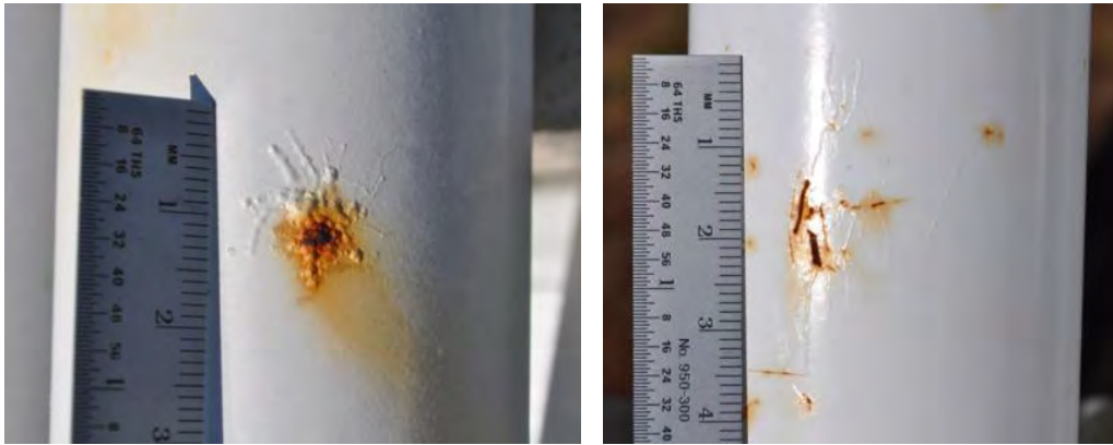
Figure 30. Coated steel railing coupon at FRF (left) and KTA (right) after 6 months of exposure.
