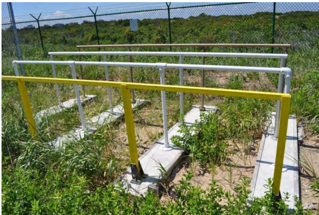
Figure 8. Railing test sections installed at the FRF.
