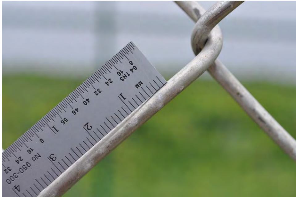
Figure B12. Aluminized Steel Wire Fencing
