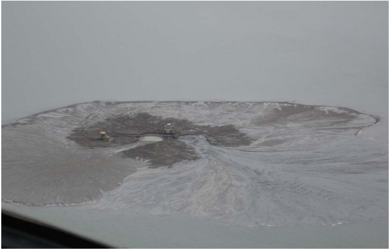
Photo 6. Aerial photo of the initial sandbar at ESH Complex 1 during construction.
