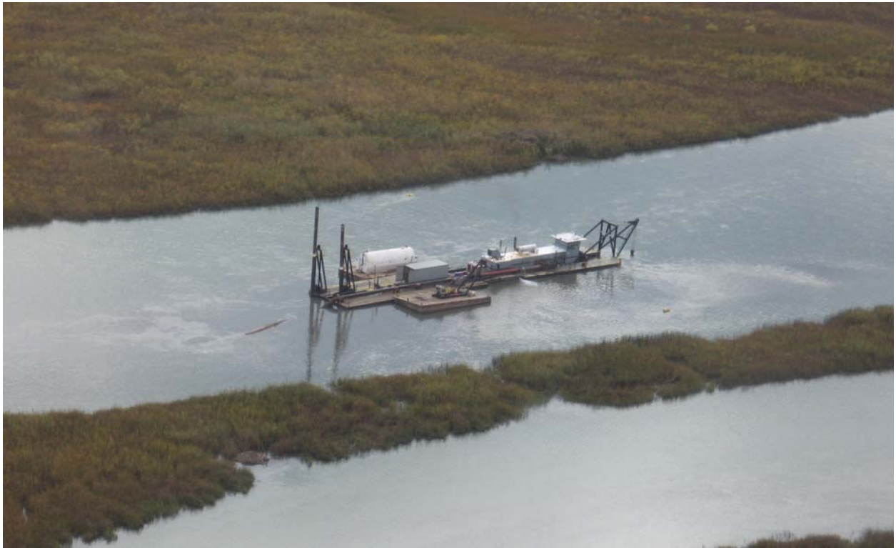
Photo 4. Aerial view of hydraulic dredge mining fill material from the initial borrow area (i.e. Borrow Area A).
