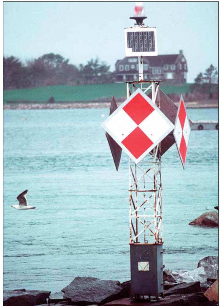
A solar-powered ATON. U.S. Coast Guard photo by Petty Officer Ron Mench.
