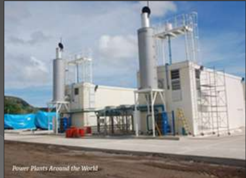
Extension to old plant
