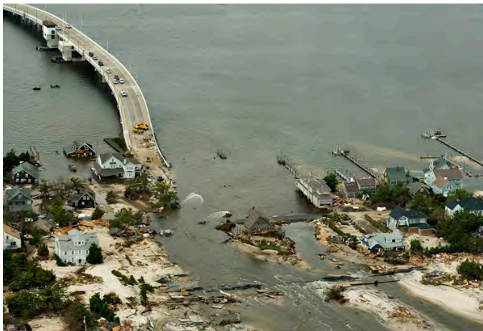
Figure 3-1. An image of the washed out Mantoloking Bridge in New Jersey after Hurricane Sandy in 2012.
