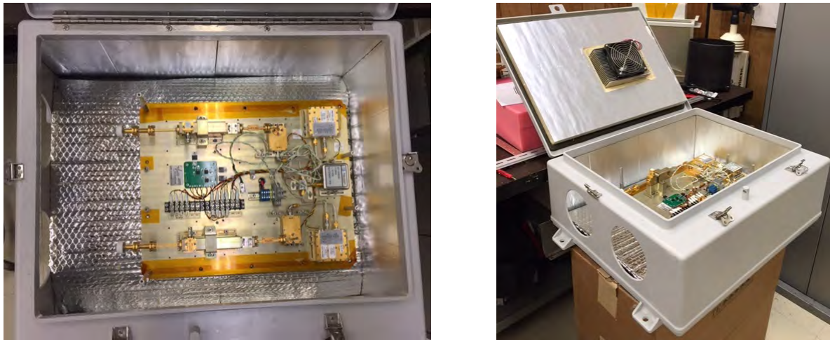
Figure 6. Transmitter Assembly in Environmentally Controlled Enclosure
