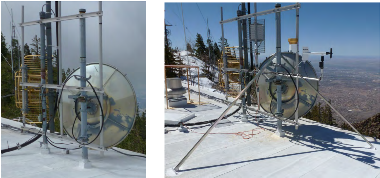
Figure 9. Fortification of WTLE Tx Antenna Mounting Structure; Before (Left) and After Brace Installation (Left)
