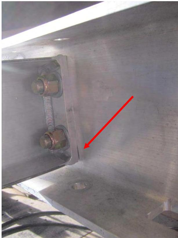
Figure 29: Damage from Half System Proof Load Test
