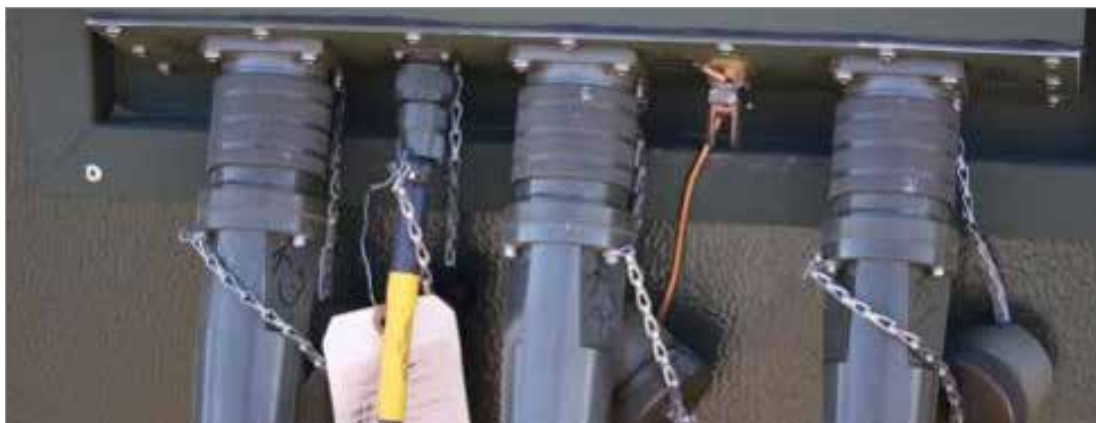
Standard MILSPEC connections for the power to the shelter from the LDSS.
