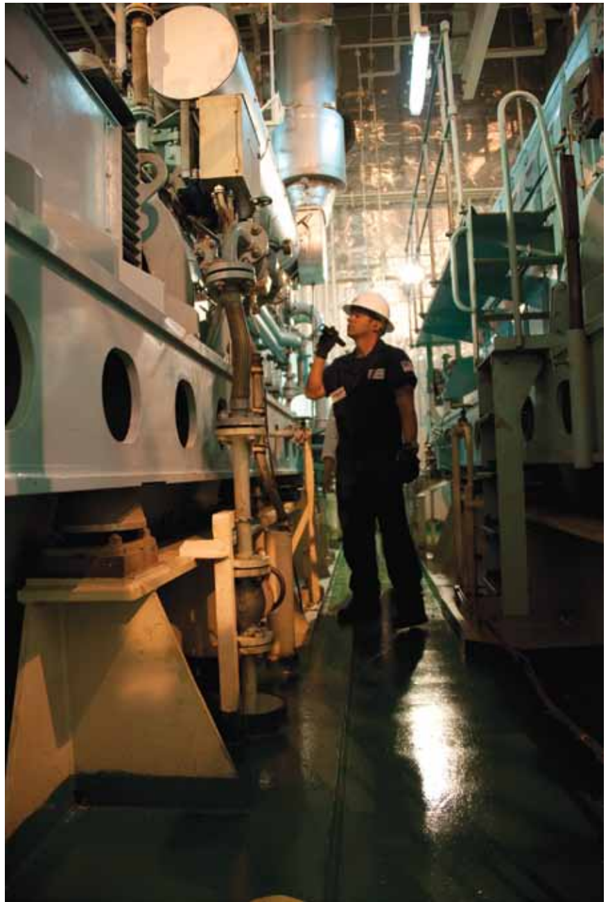
A member of U.S. Coast Guard Sector San Diego's Prevention Department inspects machinery in an engine room during an annual exam. U.S. Coast Guard photo by Petty Officer Henry G. Dunphy.
