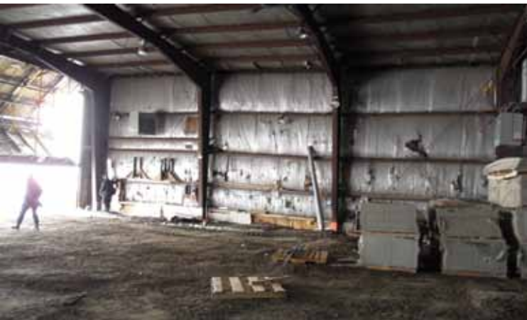
New flooring, on the pallets to the right, was instrumental to hangar upgrading. U.S. Coast Guard photo by LT Faith Reynolds.
