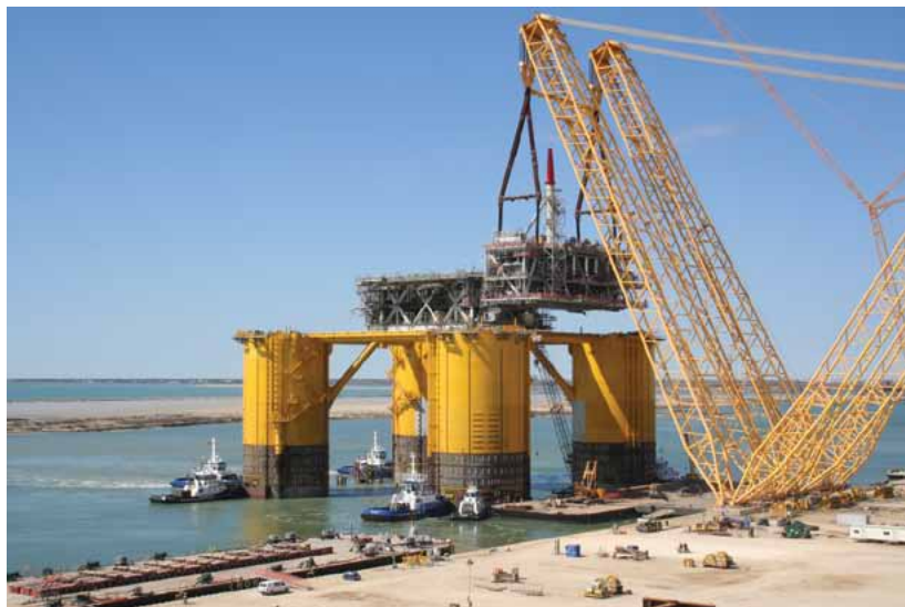
A power module is lifted onto a tension leg platform hull. U.S. Coast Guard photo by CWO Joel Smith, Sector Corpus Christi.
