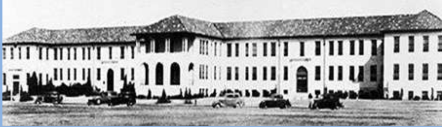
Austin Hall, Air Corps Tactical School, 1931, now Headquarters Air University
