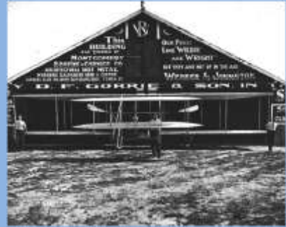
Wright Flying School Hanger and Maintenance Workshop, 1910
