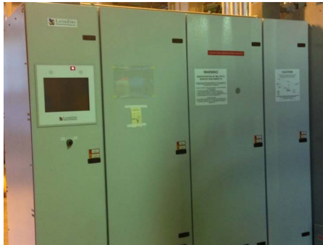
Figure 21: Microgrid Intertie Static Switch (MISS) Layer Zero
