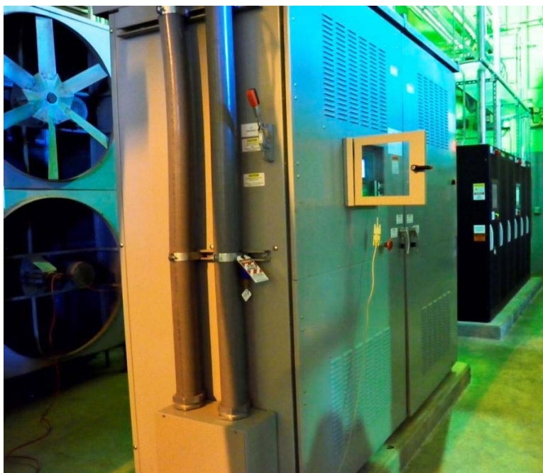
Figure 28: 500kW Storage Inverter
