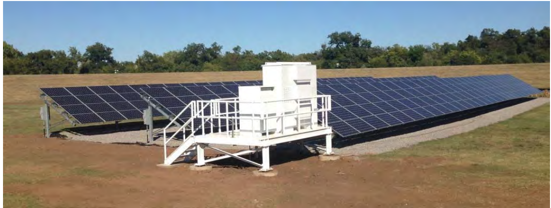
Figure 25: 86kW PV Array
