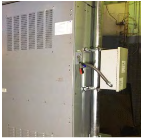
Figure 32: Storage Inverter Monitoring Unit
