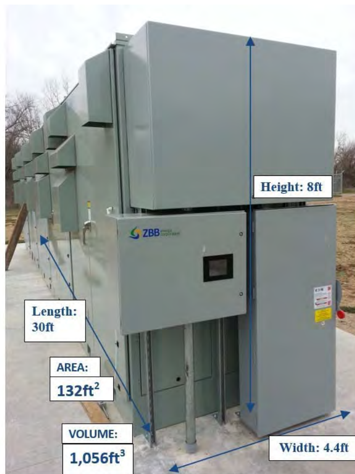
Figure 60: ZBB Flow Battery
