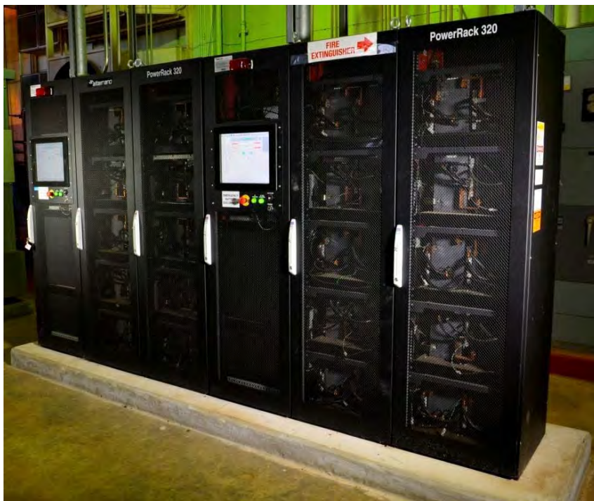
Figure 27: 400kW Power Optimized Storage Battery
