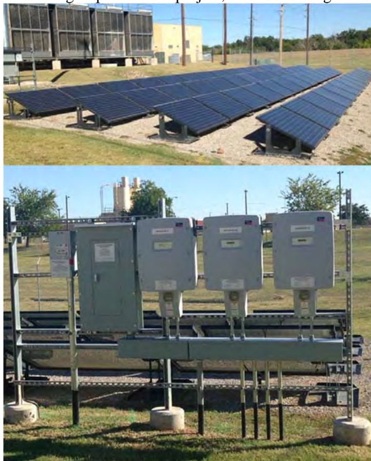
Figure 24: 17kW PV array (upper) & PV Inverters 6kW/phase (lower)
