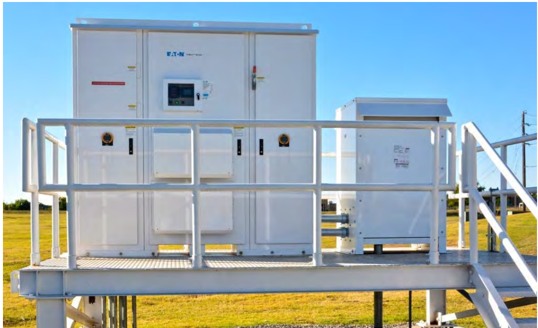
Figure 26: 86kW Array PV Inverter
