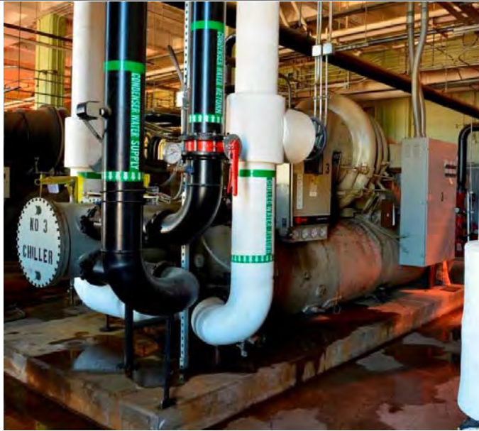
Figure 30: 350 Ton Chiller - #3
