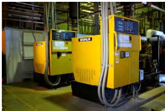
Figure 22: Caterpillar 240kW Nature Gas Generators
