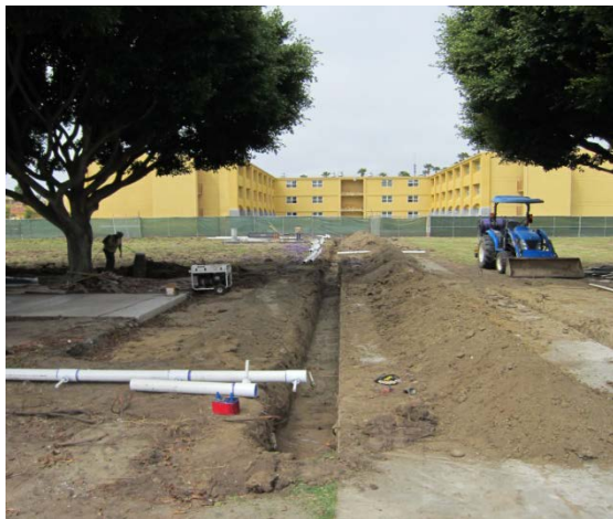
Figure 5.4. Installation of the subsurface irrigation system. Water is delivered from the clean water tank to the subsurface soil through the flexible perforated purple pipe (March 2012).
