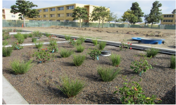
Figure 5.3. Photos of the completed installation. Filters in the LET can be removed and rinsed with a hose (left) and the treatment cells after they were planted (right) (May 2012).
