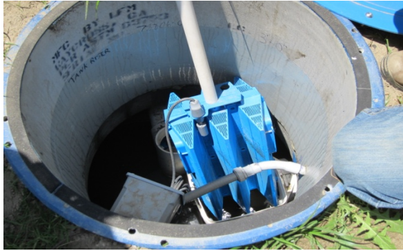
Figure 5.3. Photos of the completed installation. Filters in the LET can be removed and rinsed with a hose (left) and the treatment cells after they were planted (right) (May 2012).
