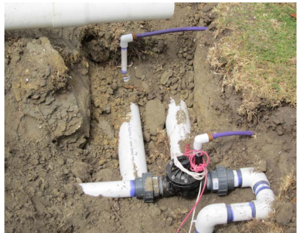
Figure 5.4. Installation of the subsurface irrigation system. Water is delivered from the clean water tank to the subsurface soil through the flexible perforated purple pipe (March 2012).
