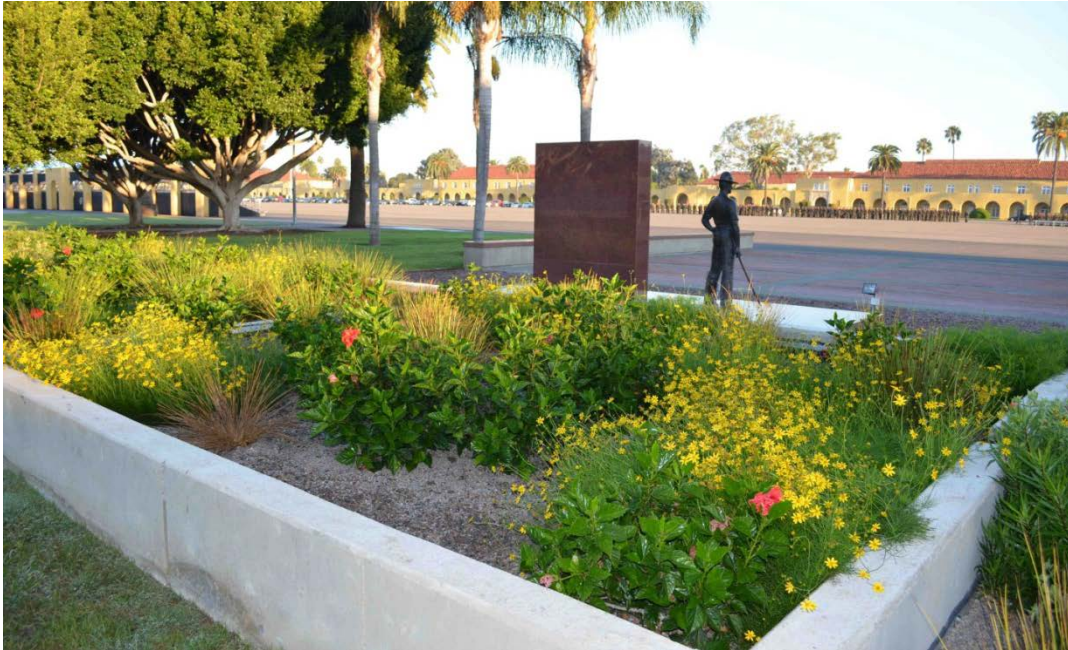
Figure 5.1. The Living Machine at MCRD with the Drill Instructors memorial in the foreground. The two center cells are the Stage 1 cells and the outermost cells are the Stage 2 cells (photo taken on 22 October 2013).
