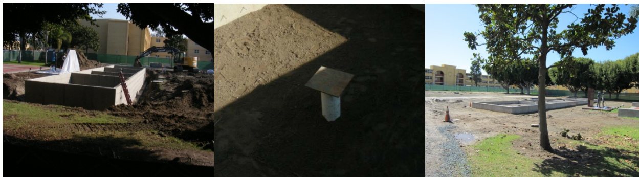
Figure 5.2. Installation of the Living Machine at MCRD showing the cast-in-place cells (left), the inlet/outlet (center) and the completed treatment cells (right). (Left and center photos December 2011; right photo February 2012).
