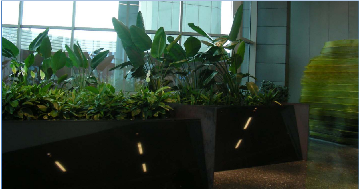
Figure 2.2. Living Machine installed in the lobby of the Portland, OR Port Authority Building (October 2011).
