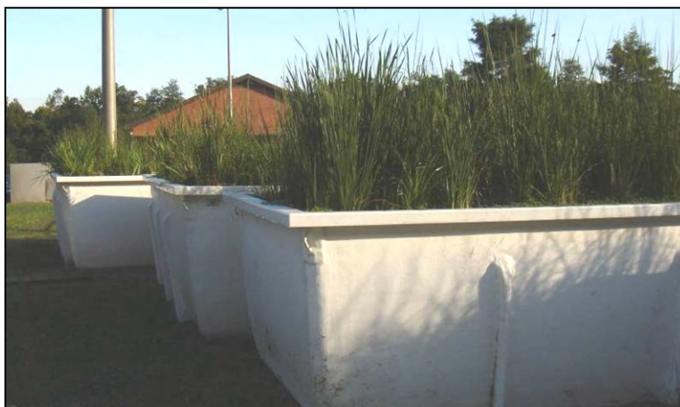
Figure 7.2. Basic and less expensive Living Machine system (with above ground tanks).
