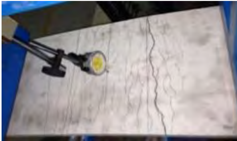
Figure 5.1 Multiple cracking of the tension face of a ferrocement panel under flexural loading ( http://www.slideshare.net/jayarawman/flexural-behaviour-of-fibre-reinforced-ferrocement-concrete ).
