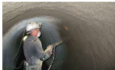
Figure 3.2 Ferrocement trowel, spray and precast production.
