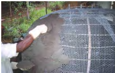
Figure 3.2 Ferrocement trowel, spray and precast production.
