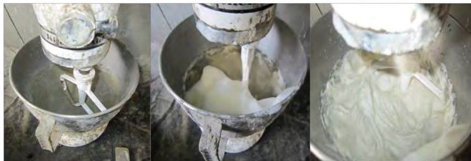
Figure 6.7 Mixing of aerated concrete.
