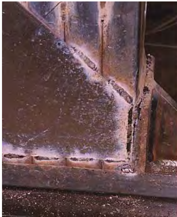
Figure 7-25. Base metal fracture of the bottom of the north column along the welded connection to the anchor.
