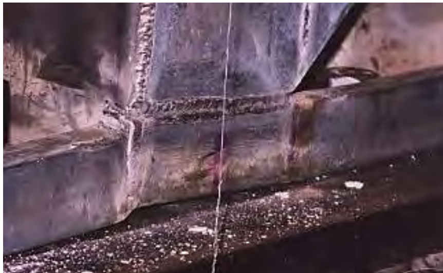
Figure 7-29. Back face of the bottom of the north column showing the pried-up and torn track at the center of the picture.
