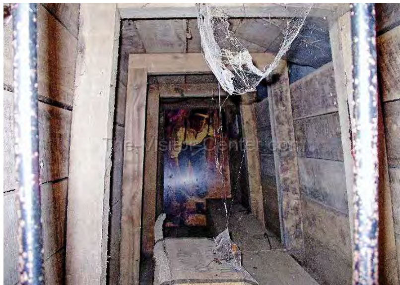
Figure 13. Inside the Union tunnel at Petersburg 41
