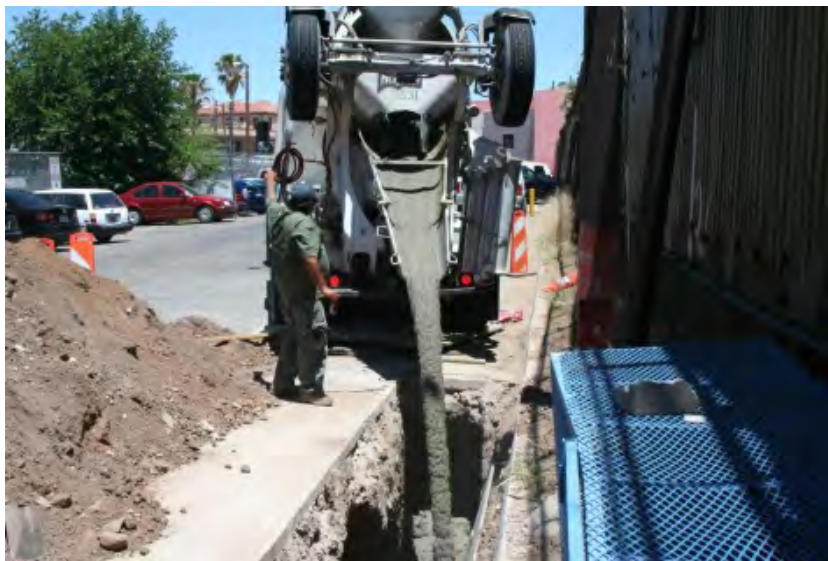
Figure 48. U.S. Customs and Border Protection Agents contract cement trucks to fill a tunnel along the Tucson sector of Nogales. 120
