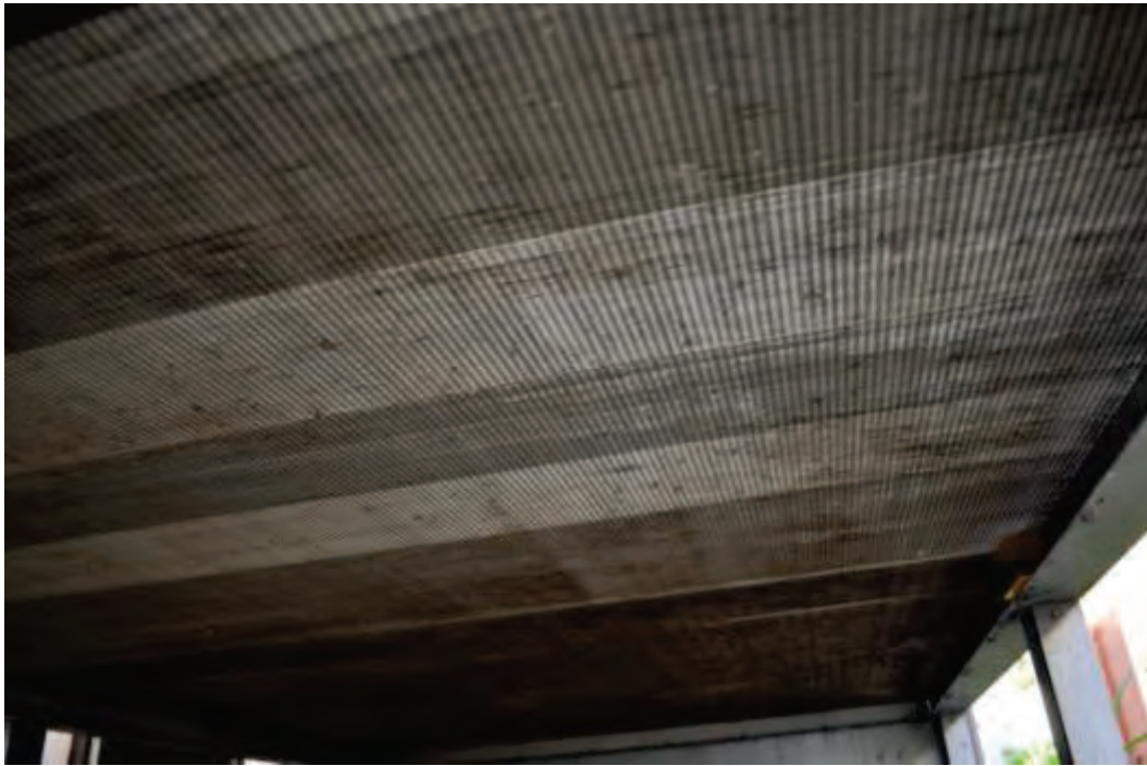
Figure A30. Coating B condenser fins at 12 months.
