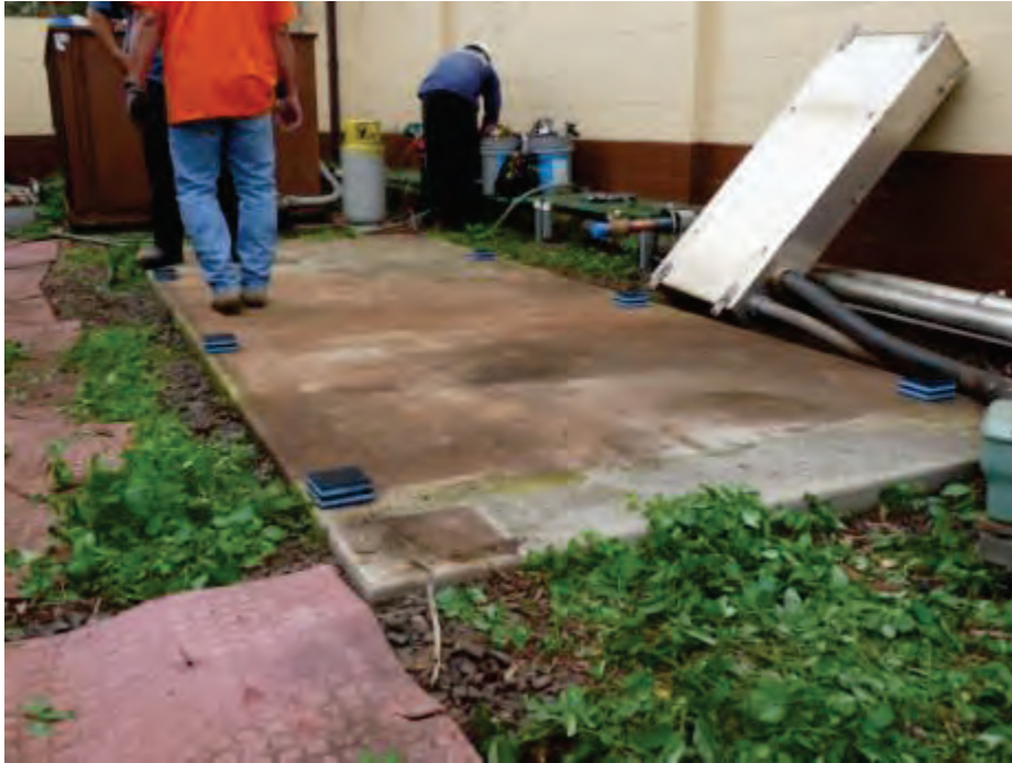
Figure 2. A condenser area cleaned of debris, with new footings in place.
