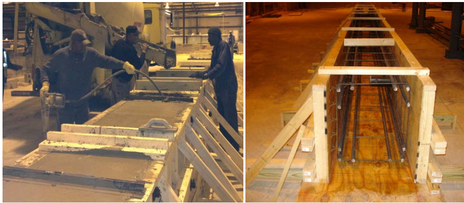
Figure 4. Full-scale 4-rod test bed during construction and concrete placement.
