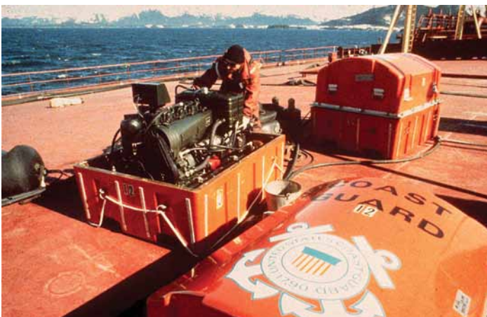
ADAPTS pumps used to lighter Exxon Valdez . U.S. Coast Guard photo.
