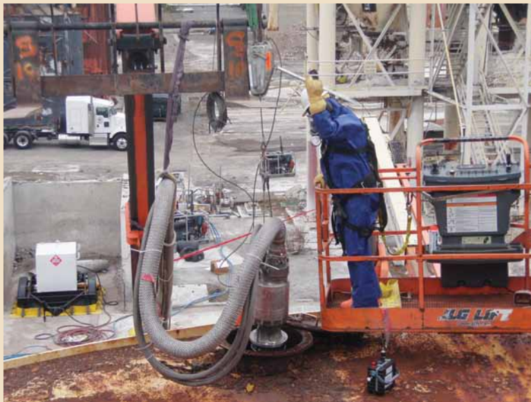
MK2 Jeffrey Burby, Pacific Strike Team, lowers a chemical-resistant pump into a degraded tank. U.S. Coast Guard photos by MKC Travis Olson.
