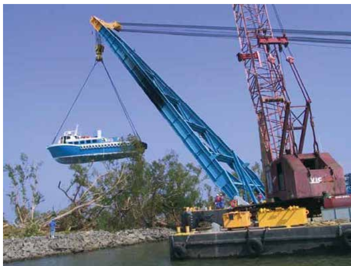
Post-hurricane response salvage and heavy lift operation. Photos courtesy of T&T Marine Salvage.
