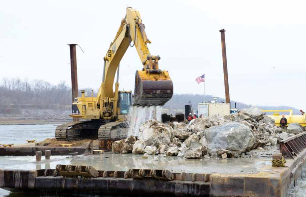
Crews work to remove the rocky obstructions during the low water operations near Thebes, Ill., in 2012. Photo courtesy of the U.S. Army Corps of Engineers, St. Louis District-MVS, photo by Romanda Walker.
